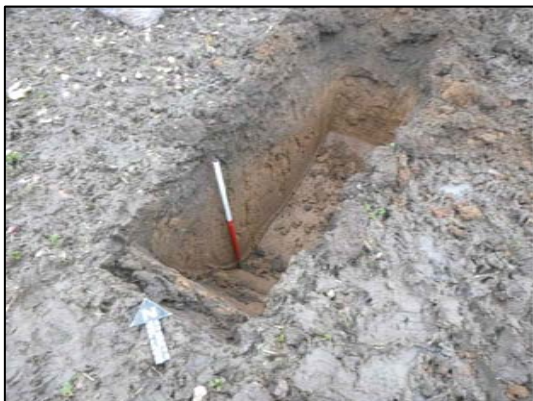
CBR 7, looking north
