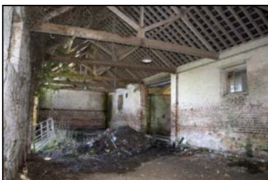
GIL18-0028 Interior of the barn. Facing south-west
