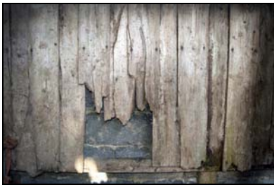
GIL18-0079 Weatherboard section of dairy. Facing north
