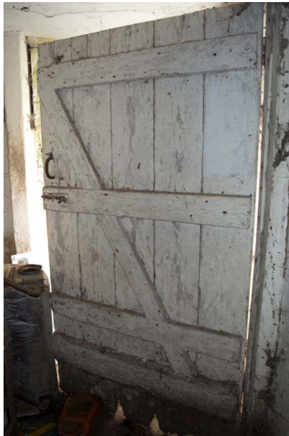
Plate 33 – Boarded and braced door in the dairy, facing east (GIL18-0087)
