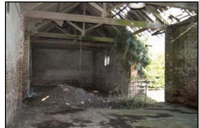
GIL18-0042 Interior of the barn. Facing north-east
