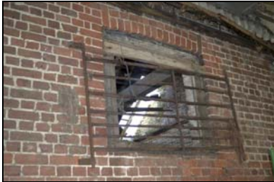
GIL18-0022 Detail of the inserted window. Facing south-east
