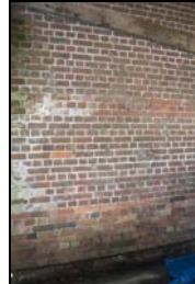
GIL18-0020 Detail of the brickwork, west facing elevation. Facing east
