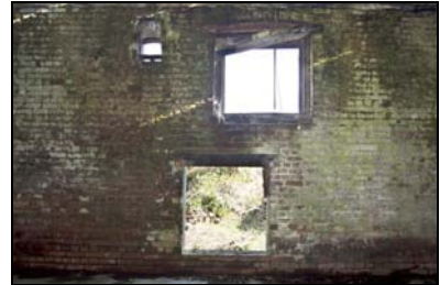
GIL18-0039 Inserted openings. Facing east
