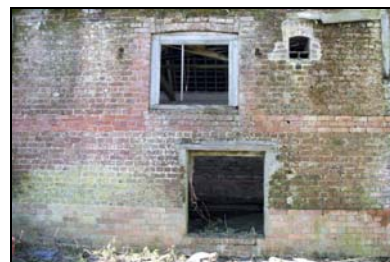
GIL18-0006 Inserted openings in the east facing elevation. Facing west
