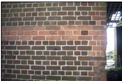
GIL18-0025 Plat band detail on the west facing elevation. Facing east
