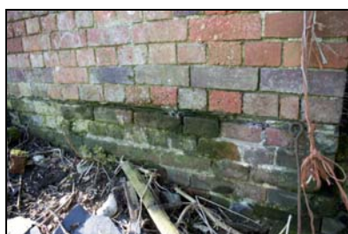
GIL18-0010 Detail of the brickwork showing damp proof coursing. Facing south-west
