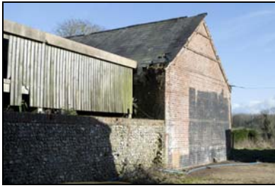
GIL18-0016 South facing gable end and yard wall. Facing north-east
