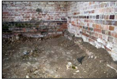
GIL18-0032 Detail of the differing brickwork. Facing west
