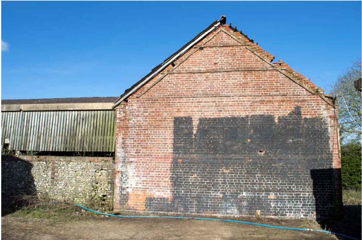
Plate 5 – The south gable of the barn, facing north (GIL18-0015)
