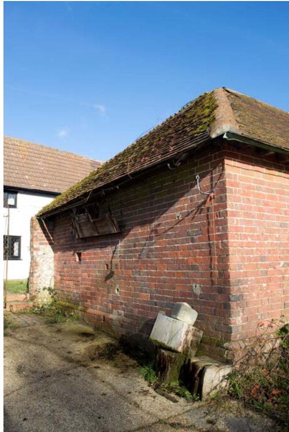
Plate 19 – The western end of the dairy, facing north-east (GIL18-0069)
