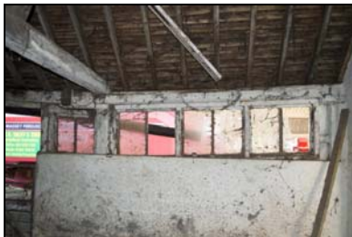
GIL18-0101 Inserted windows in the weatherboard wall. Facing south
