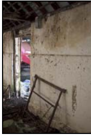
GIL18-0094 Detail of rendered walls in the dairy. Facing south-east
