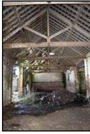
GIL18-0031 Interior of the barn. Facing south
