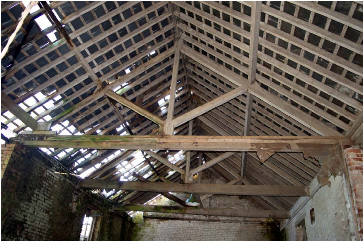
Plate 9 – Roof truss construction in the barn, facing south (GIL18-0058)
