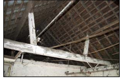
GIL18-0093 Detail of roof trusses in the dairy
