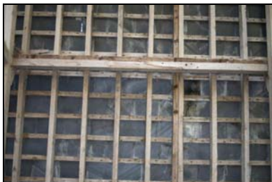
GIL18-0049 Detail of the rafters. Facing east
