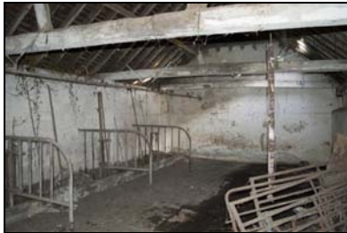
GIL18-0098 Interior of the dairy, room four. Facing north-east
