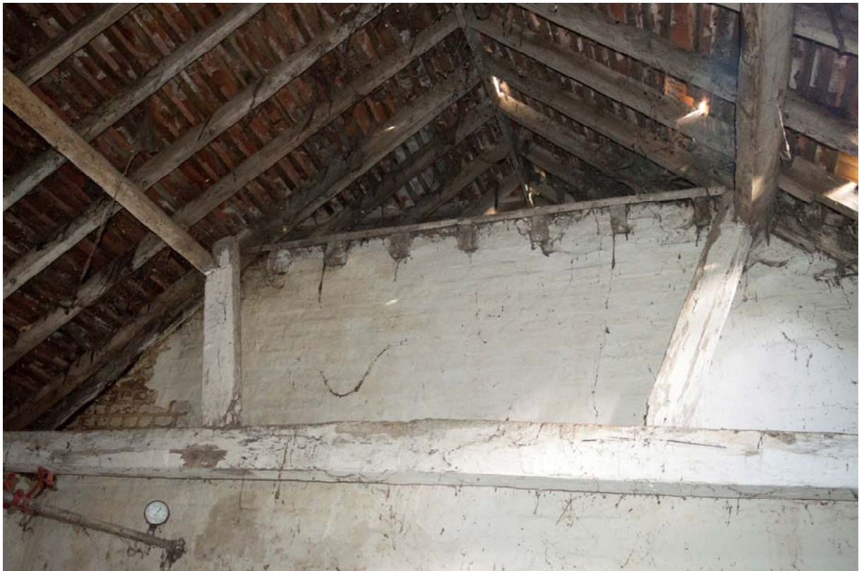
Plate 29 – Truss positioned just before the barn wall inside the dairy, facing north-east (GIL18-0110)
