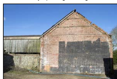
GIL18-0015 South facing gable end. Facing north
