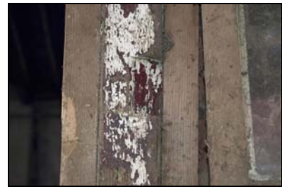
GIL18-0081 Detail of notch in weatherboard framing. Facing north
