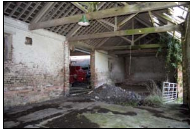
GIL18-0044 Interior of the barn. Facing north-west
