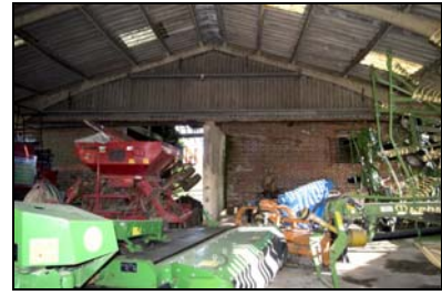
GIL18-0018 The barn, west facing elevation. Facing east
