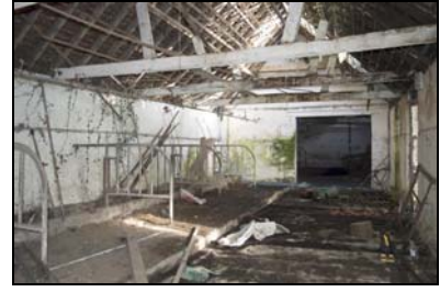
GIL18-0090 Interior of the dairy room three. Facing north-east
