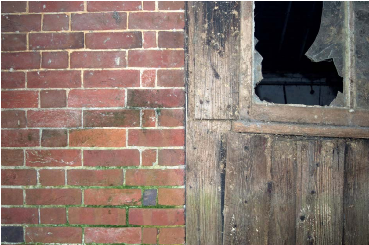
Plate 22 – Junction of the brickwork and weatherboarding showing queen closer bricks, facing north (GIL18-0077)
