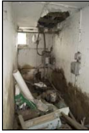
GIL18-0088 Interior of the dairy, room two. Facing north
