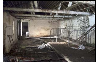
GIL18-0096 Interior of the dairy room three. Facing west
