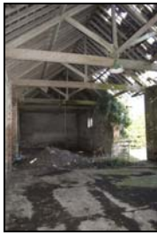
GIL18-0043 Interior of the barn. Facing north-east
