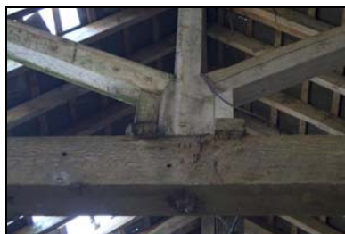
GIL18-0053 Detail of carpenters marks
