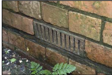
GIL18-0023 Detail of a cast iron ventilation block. Facing north-east
