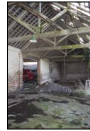
GIL18-0045 Interior of the barn. Facing north-west
