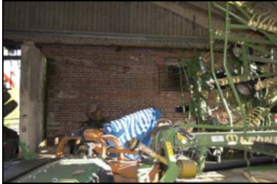
GIL18-0019 The barn, west facing elevation. Facing east
