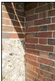
GIL18-0067 Detail of dairy wall and yard wall. Facing north
