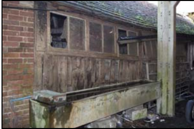
GIL18-0076 South facing elevation of the dairy. Facing north
