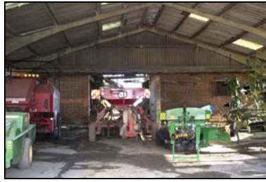
GIL18-0017 The barn, west facing elevation. Facing east
