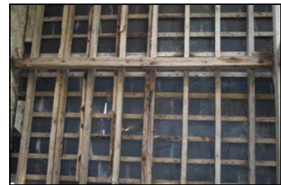
GIL18-0048 Detail of the rafters in the southernmost bay. Facing east
