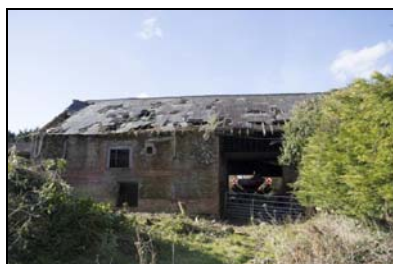
GIL18-0001 The barn, east facing elevation. Facing west
