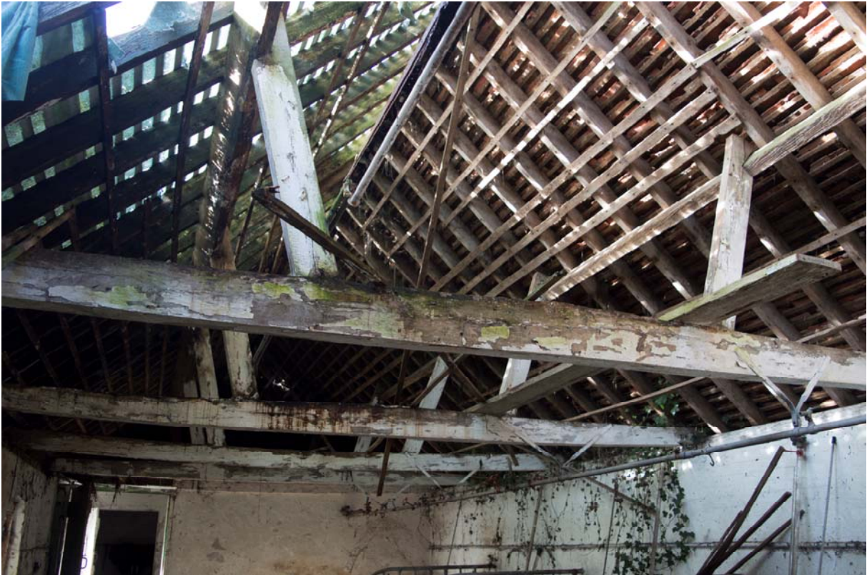
Plate 27 – The roof of the dairy, facing north-west(GIL18-0097)
