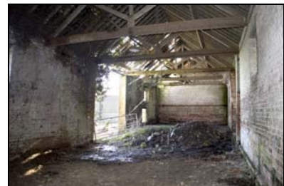
GIL18-0027 Interior of the barn. Facing south-east
