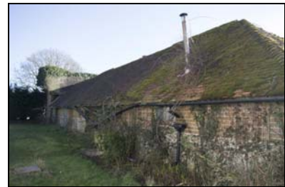
GIL18-0066 North facing elevation of the dairy. Facing south-east
