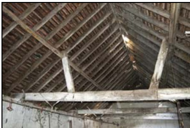
GIL18-0100 Detail of the roof structure, room four
