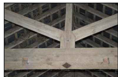
GIL18-0057 Detail of carpenters marks
