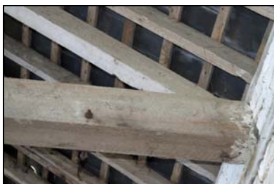
GIL18-0052 Detail of carpenters marks
