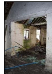
GIL18-0102 Inserted opening between rooms three and four. Facing south-west
