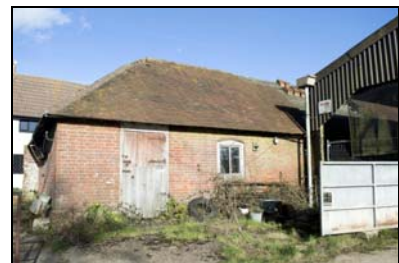
GIL18-0072 South facing elevation of the dairy. Facing north
