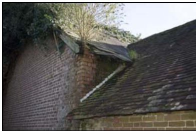
GIL18-0064 Join of the barn and dairy roofing. Facing south-east
