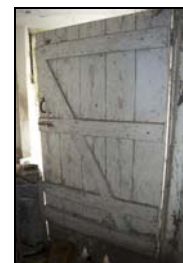
GIL18-0087 Board and brace door inside the dairy. Facing east
