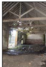
GIL18-0026 Interior of the barn. Facing south-east
