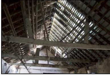
GIL18-0092 Detail of the roof structure in the dairy
