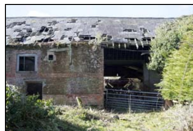
GIL18-0003 The barn, east facing elevation. Facing west
