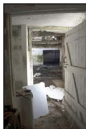
GIL18-0086 Interior of the dairy. Facing east
