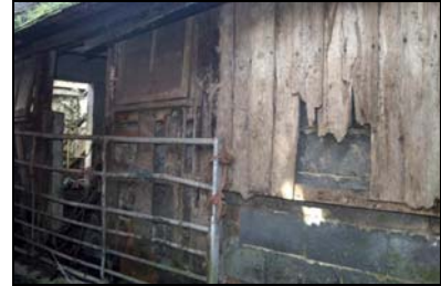
GIL18-0078 Weatherboard section of dairy. Facing north-west
