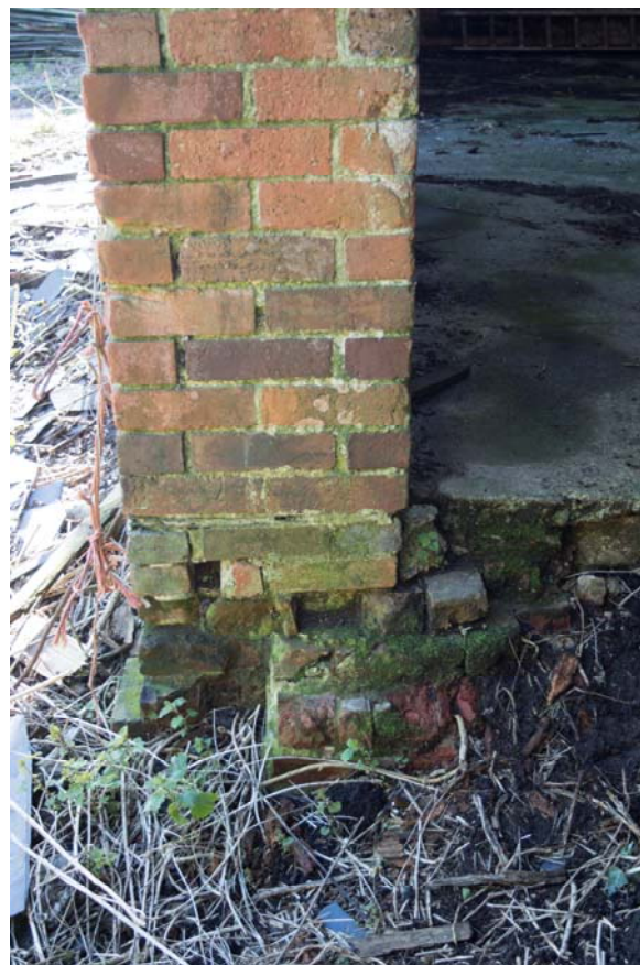
Plate 8 – Truncated earlier brickwork visible at the midstrey opening, facing south (GIL18-0012)
