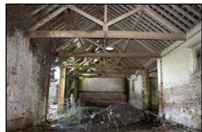
GIL18-0030 Interior of the barn. Facing south
