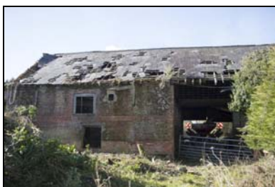
GIL18-0002 The barn, east facing elevation. Facing west
