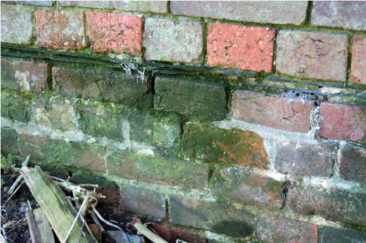
Plate 7 – Earlier brickwork below the slate damp-proof course, facing south-west (GIL18-0011)
