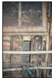
GIL18-0080 Weatherboard section of dairy. Facing north
