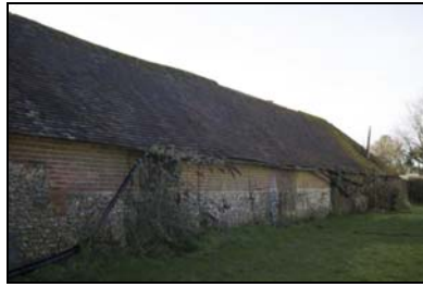
GIL18-0062 North facing elevation of the dairy. Facing south-west
