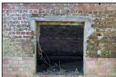
GIL18-0007 Detail of the lower inserted opening. Facing west
