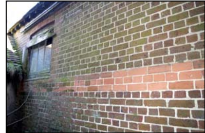
GIL18-0024 West facing elevation. Facing north-east
