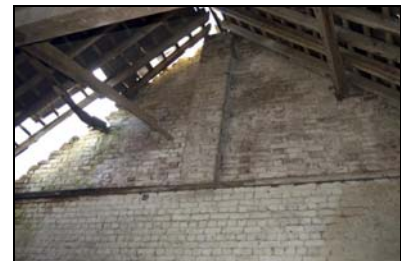
GIL18-0051 Detail of the interior of the southern gable. Facing south-east
