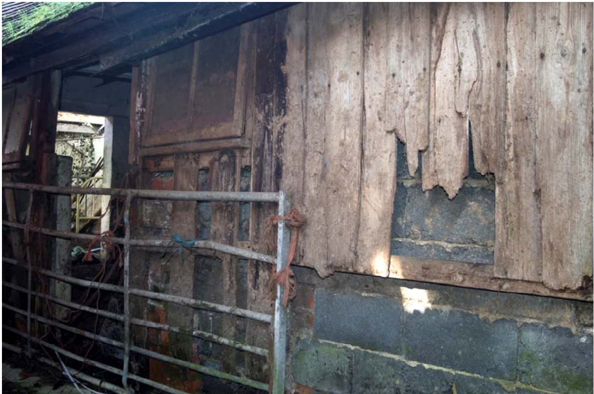
Plate 21 – Boarded eastern end of the dairy, facing north-west (GIL18-0078)
