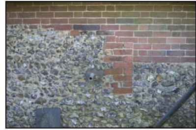
GIL18-0063 Detail of the flint walling. Facing south
