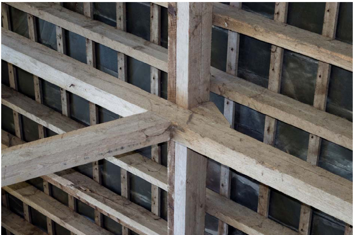
Plate 10 – Detail of roof construction, facing south (GIL18-0050)
