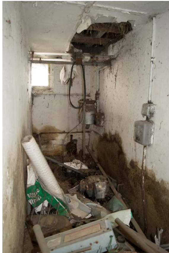
Plate 32 – Room 2 of the dairy, facing north (GIL18-0089)
