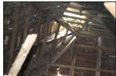
GIL18-0084 Detail of the the hipped roof structure
