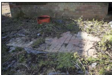
GIL18-0005 Brick paving outside the barn. Facing south-west
