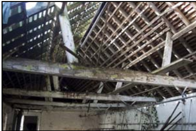
GIL18-0097 Detail of the roof structure, room three
