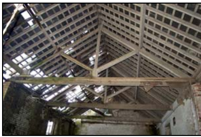
GIL18-0058 Detail of the roof truss structure
