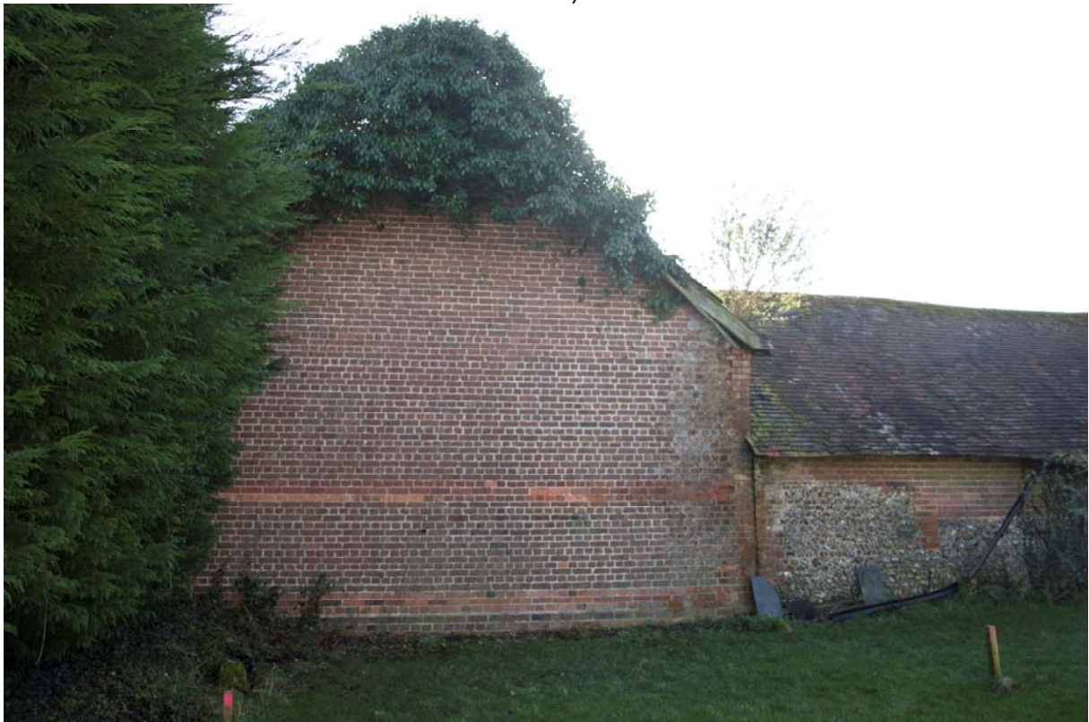
Plate 4 – The north gable of the barn, facing south (GIL18-0059)
