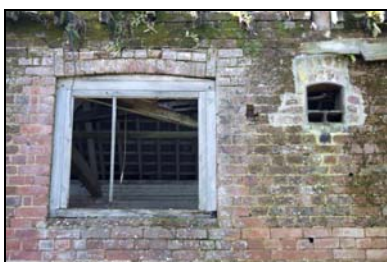
GIL18-0008 Detail of the high-set inserted openings. Facing west
