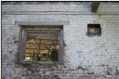
GIL18-0040 Inserted openings. Facing west
