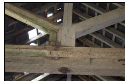
GIL18-0054 Detail of carpenters marks
