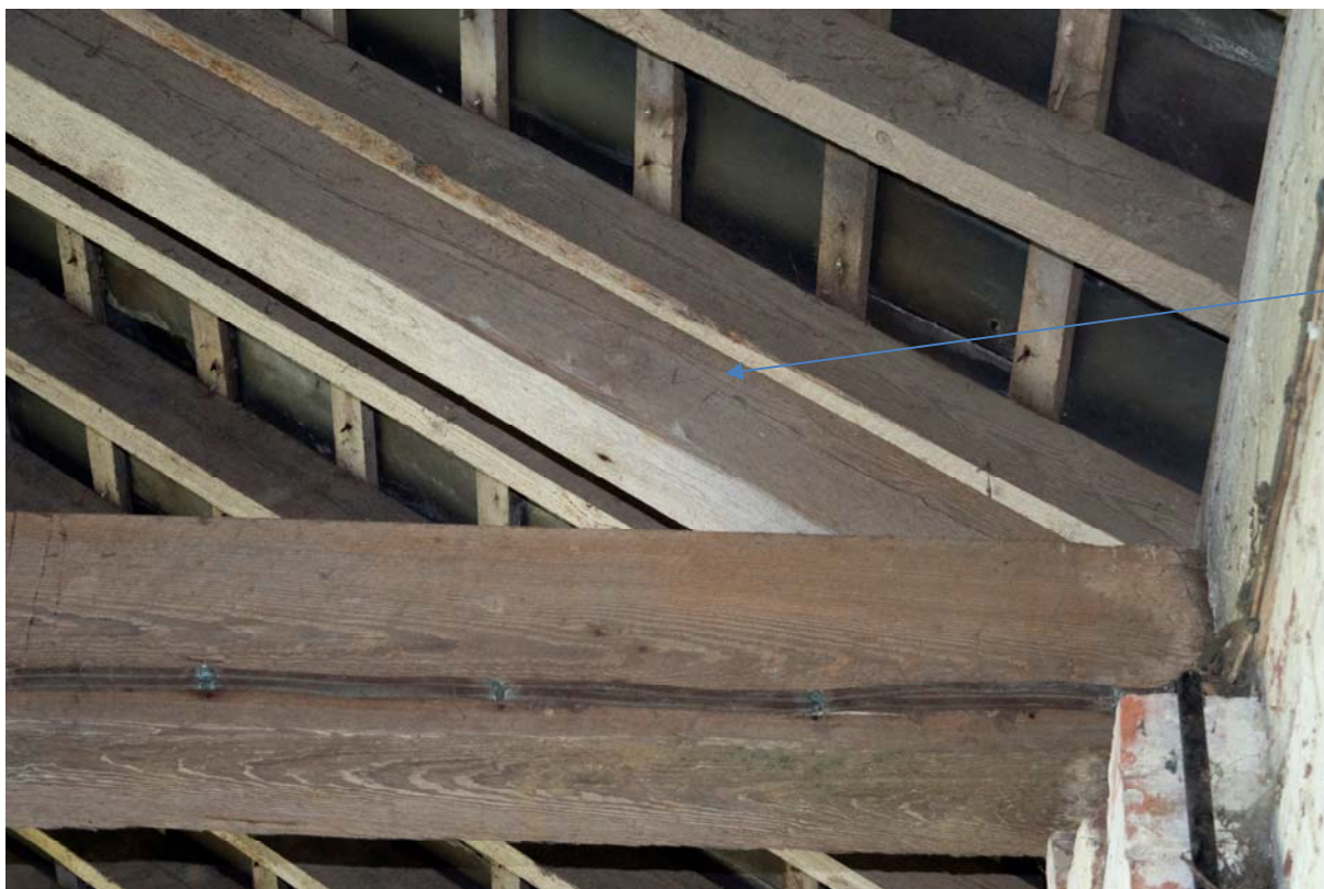
Plate 12 – Examples of carpentry marks on trusses in the barn, facing south (GIL18-0055)
