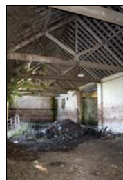
GIL18-0029 Interior of the barn. Facing south-west
