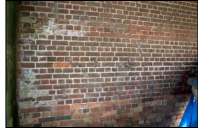
GIL18-0021 Detail of the brickwork, west facing elevation. Facing east
