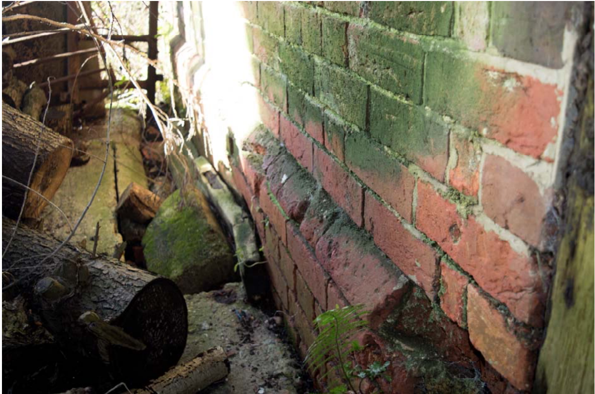
Plate 23 – Brick offset at the base of the dairy walls, facing north-west (GIL18-0082)
