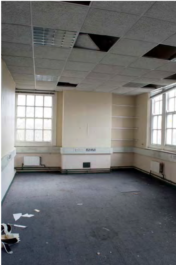
Plate 19: Removal of the officers' bedrooms has created office space (SJH18-0106)
