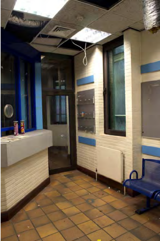
Plate 13: Former Inspector's office, now reception area (SJH18-0042)
