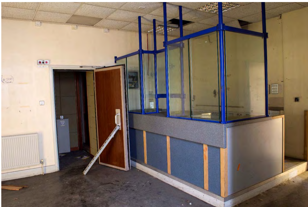
Plate 12: Charge room with inserted booth (SJH18-0044)
