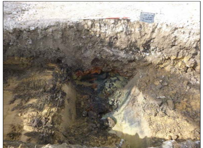
Trench 4 test pit looking South-West
