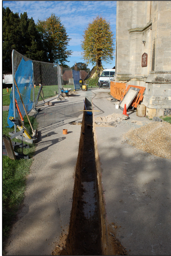
View north along the pipe trench from the manhole
