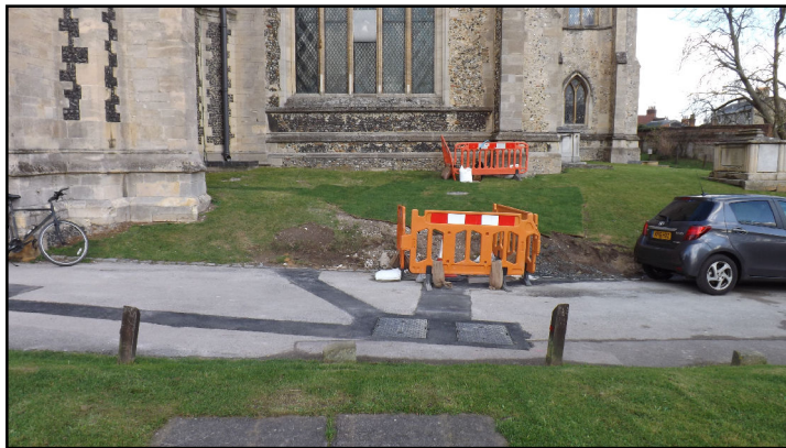
View west to the South Aisle showing bank
