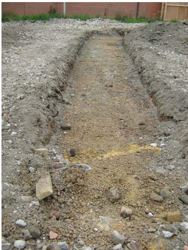
Plate 4: Trench 3 looking west
