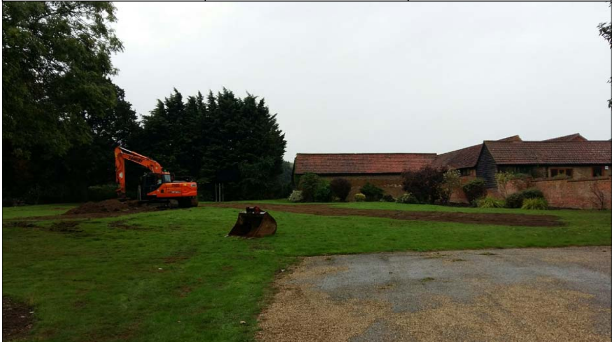
General site view
