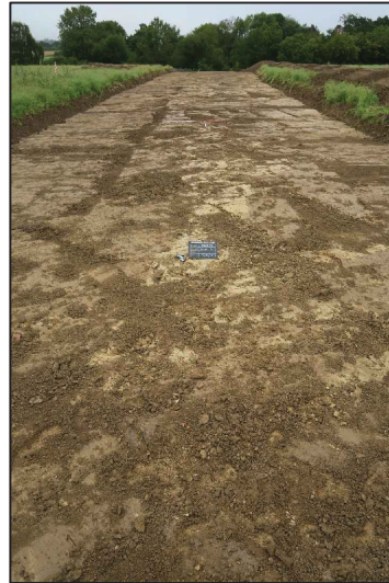
Area A, looking north east
