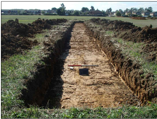
Trench 11, looking south west
