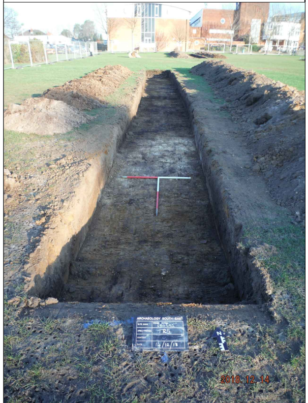
Trench 5 facing north
