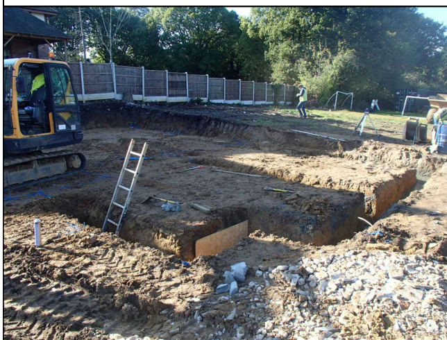
Plot 3 foundation trenches
