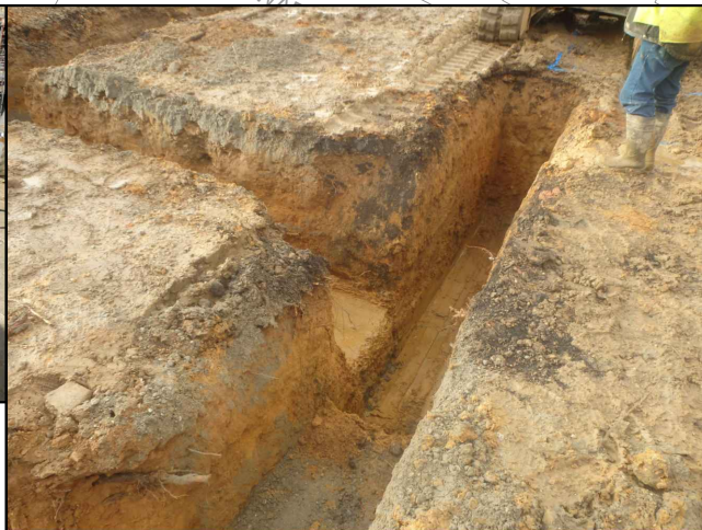
Plot 2 foundation trenches
