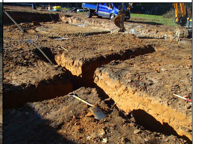
Plot 4 foundation trenches
