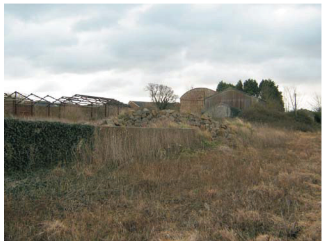
Plate 4: Concrete wall of animal yard, facing SE
