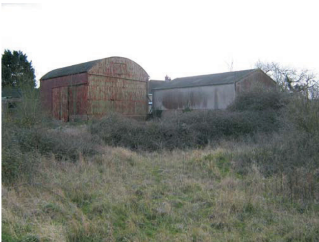
Plate 5: General shot of farmyard barns due for demolition, facing SW
