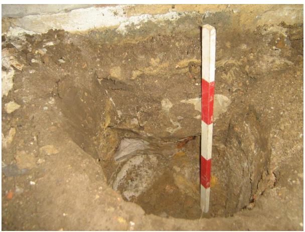
Plate 4: Wall footing below north wall of potting shed, from inside shed
