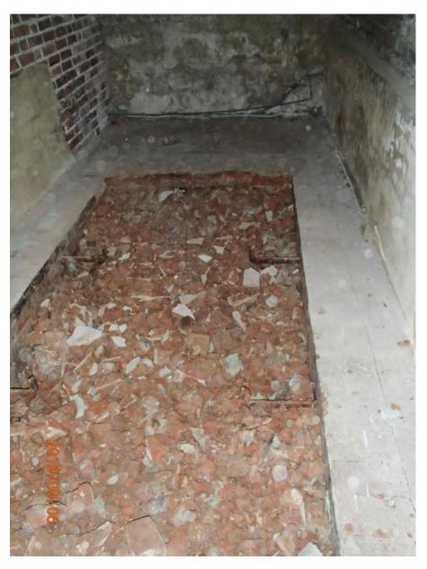
Plate 23: Hardcore beneath the concrete floor at the east end of the Wagon Lodge
