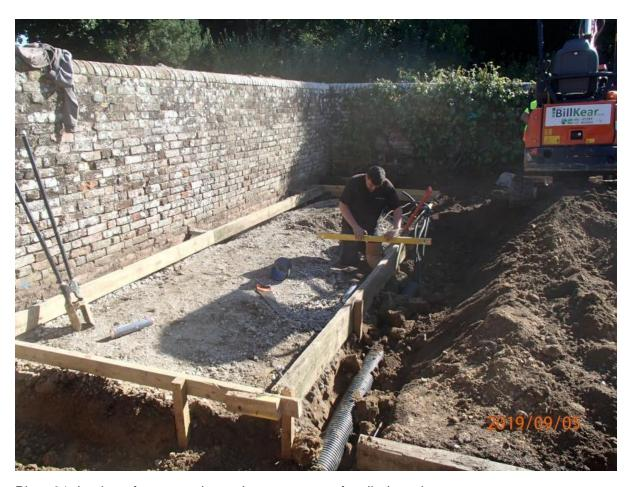
Plate 31: Laying of concrete in north-east corner of walled garden
