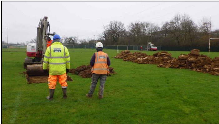
Excavation of Trench 5 (foreground) and Trench 7 (background)
