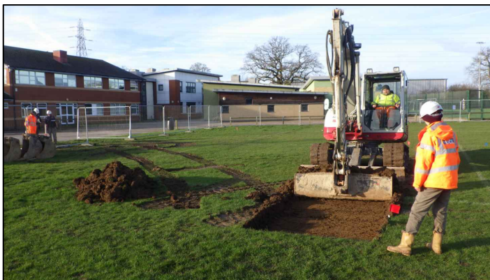
Excavation of Trench 10
