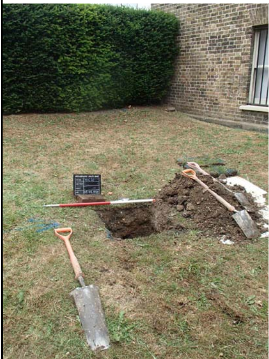
Sondage in relation to Milton Chantry Heritage Centre looking North-West
