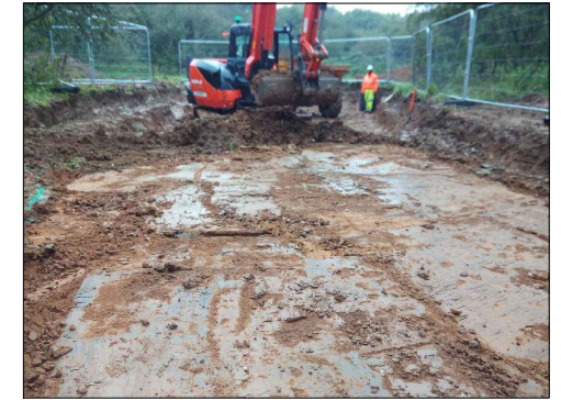
Ground reduction of badger sett, looking west
