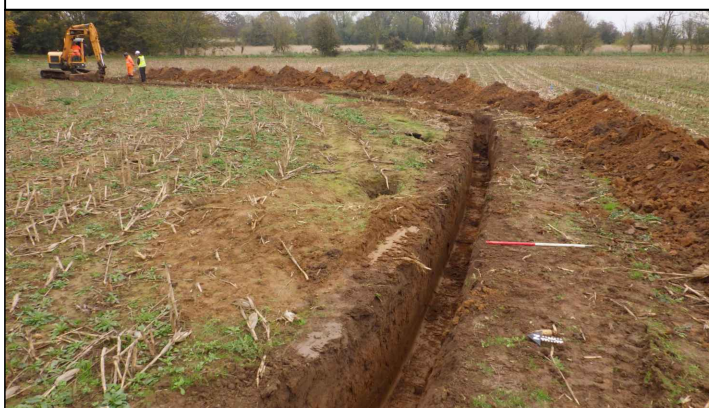
Trench for badger netting, looking east
