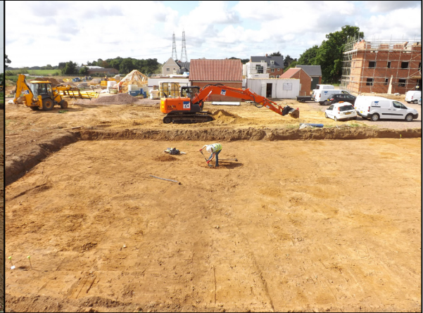
PH2. The site during excavations
