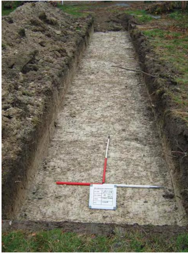
© Archaeology South-East Well Road, Otford Fig. 12 Project Ref: 3324 June 2008 Trench 15 (South-south-west facing) Report Ref: 2008065 Drawn by: SM
