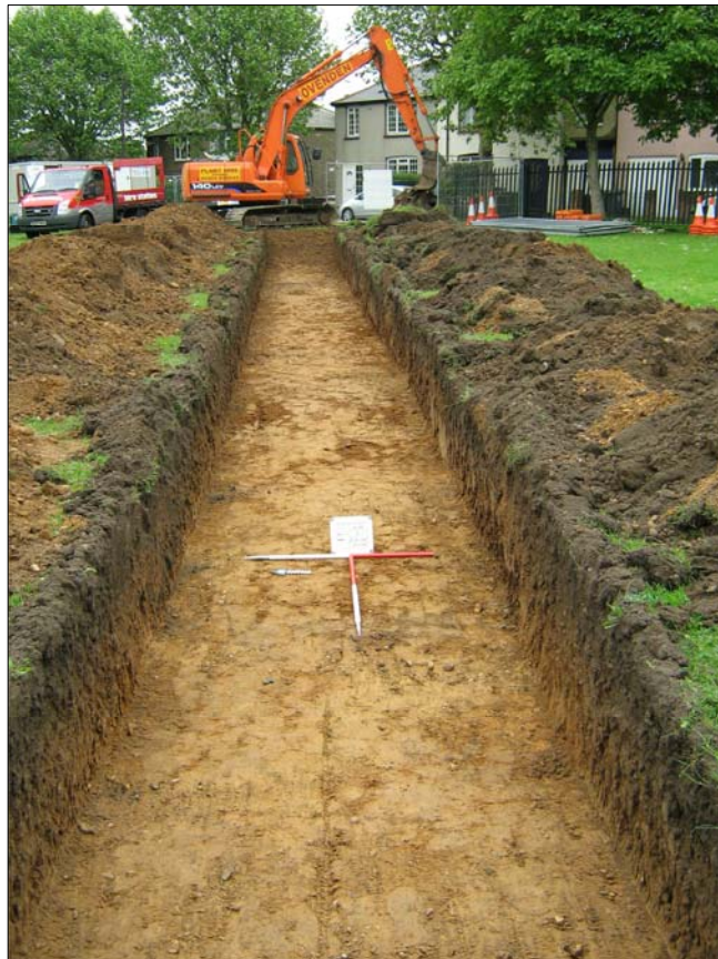
Fig. 4: Trench 1 looking east
