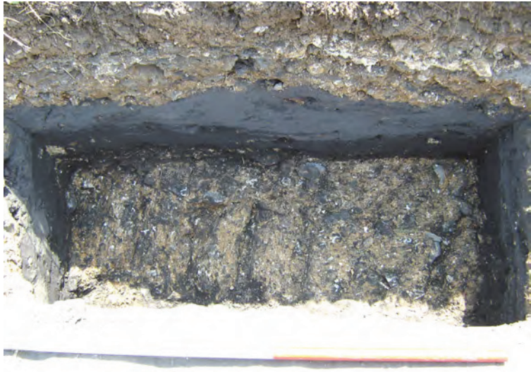
Fig. 7: Photo highlighting potential mechanical excavator tracks within trench 2
