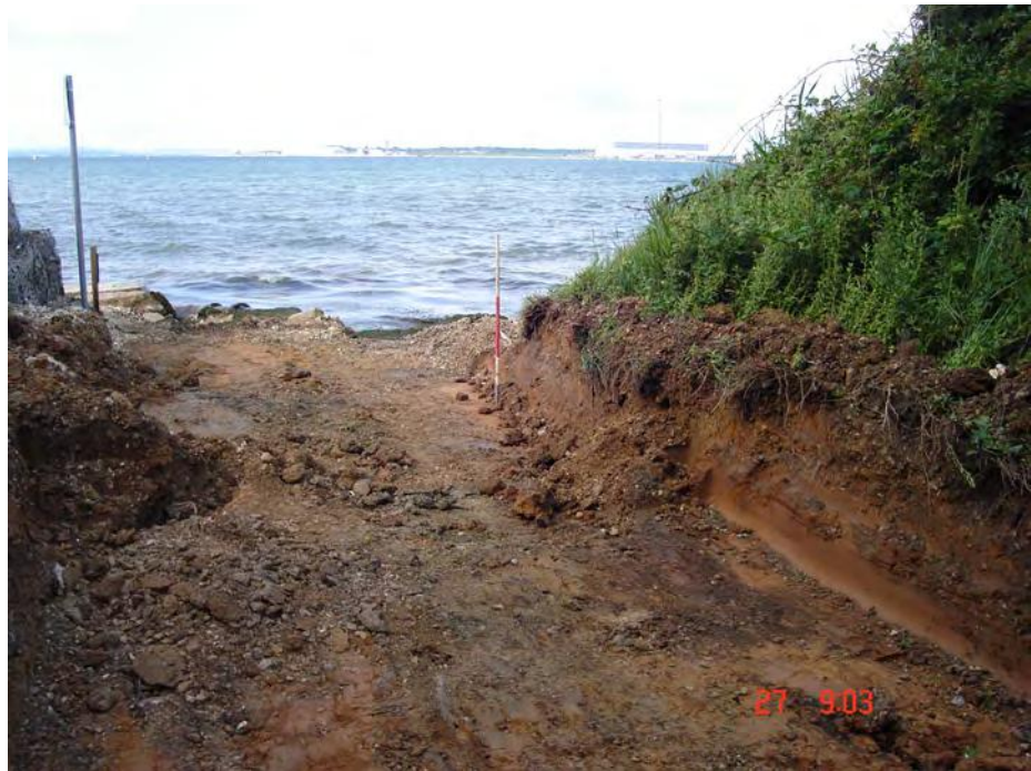
Fig. 5: General shot of easement corridor looking south
