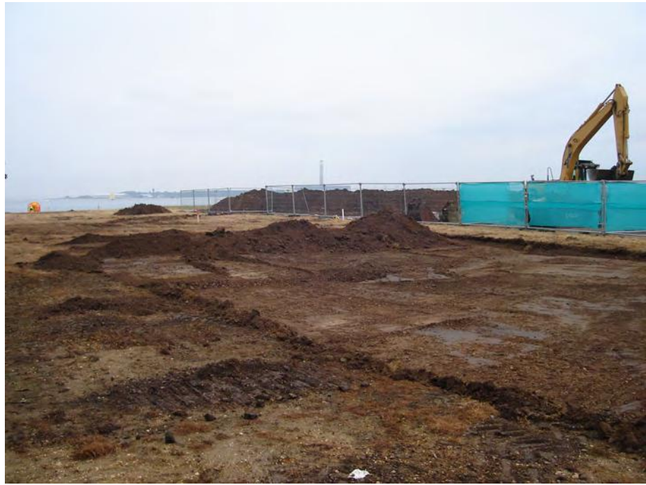
Fig. 4: General shot of easement corridor looking south-west
