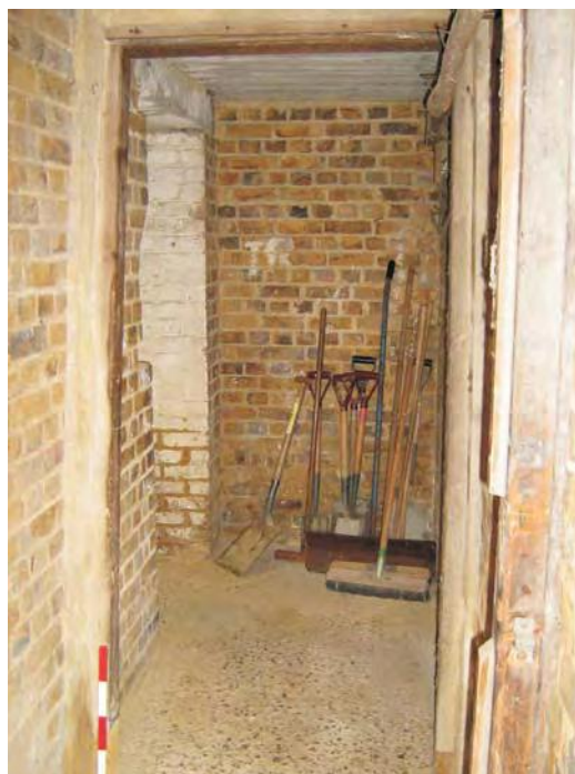
Plate 4: The south traverse passage with diagonal housing for additional blast-protection doorway
