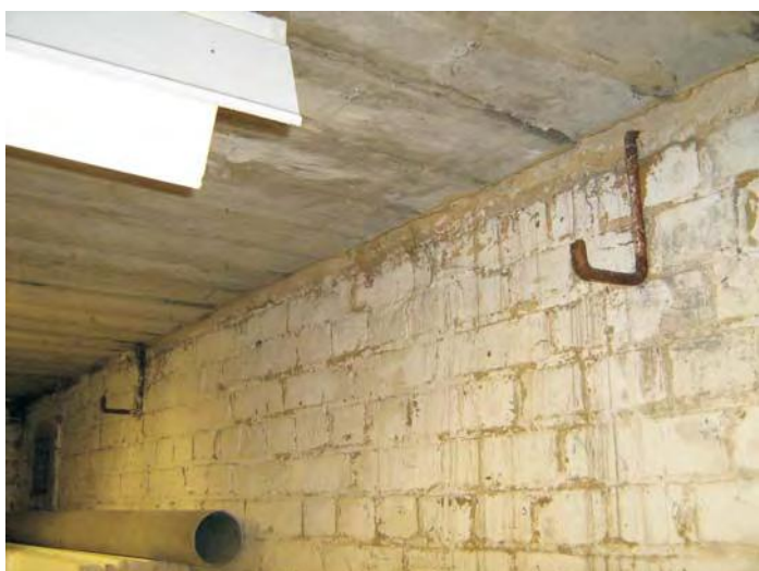
Plate 5: Detail of the shuttered concrete roof in the interior of the south room, shows whitewashed walls and hooks
