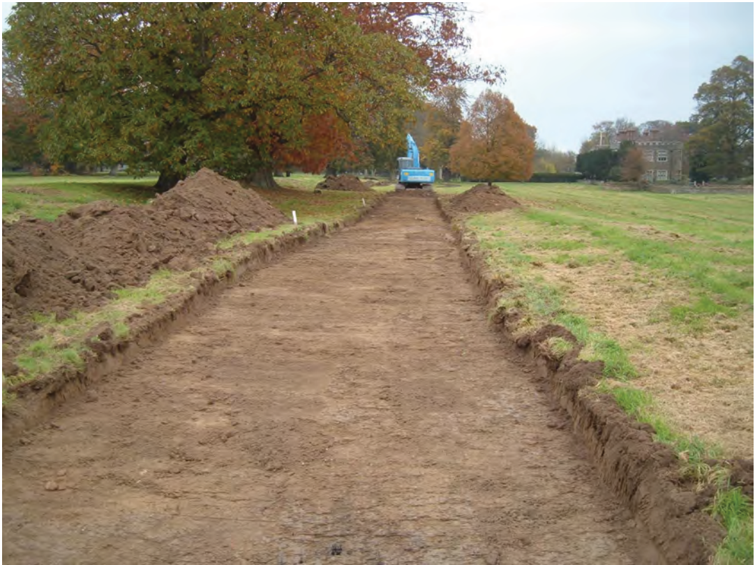
Fig. 5: Photograph of driveway excavation in progress (looking north)
