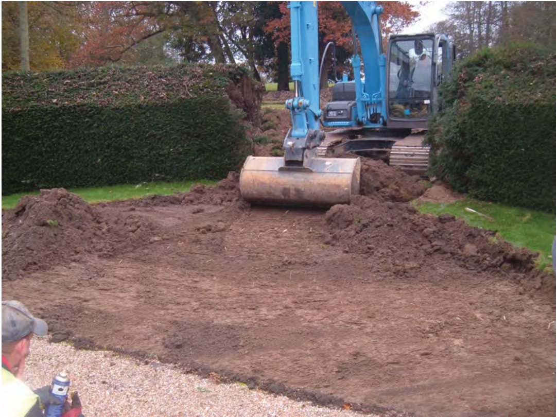
Fig. 4: Photograph of driveway excavation looking east showing deposit [106]
