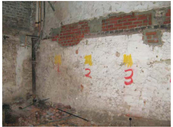
Arch junction with brickwork extending up to former ceiling level
