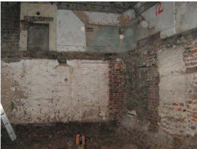
Plate 11: The west wall with unpainted brick feature to the north
