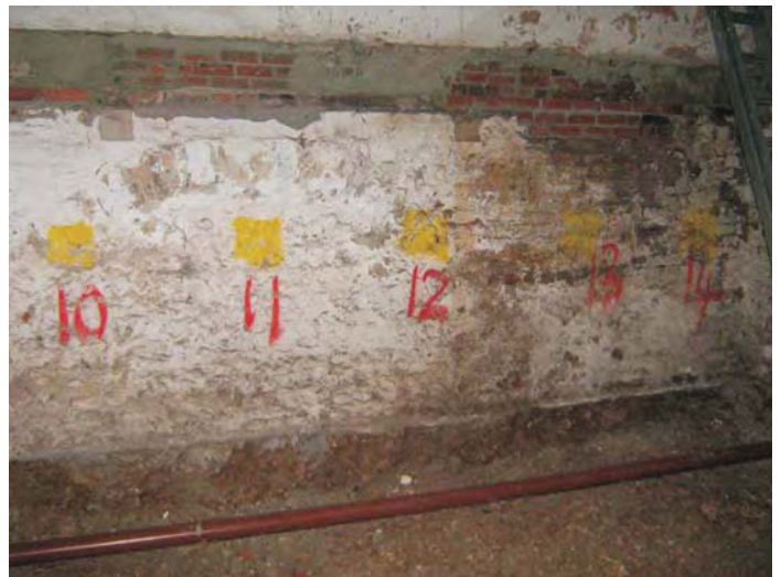
Plate 8: The painted south elevation
