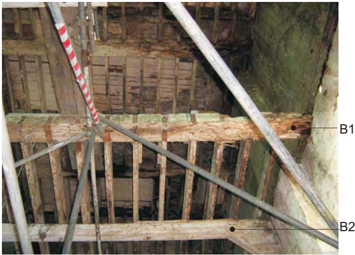
Plate 13: Remnant ceiling construction at First Floor
