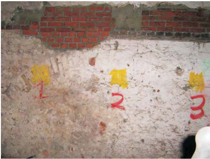
Plate 9: Detail of an arch in the south wall
