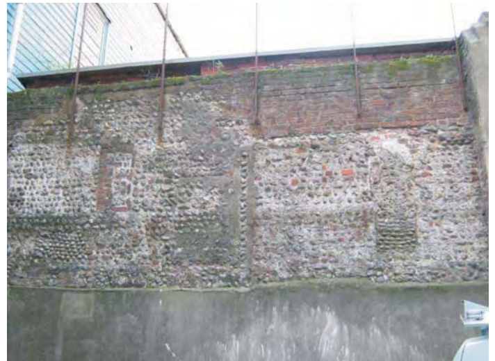
Plate 16 : The west perimeter wall in the car park
