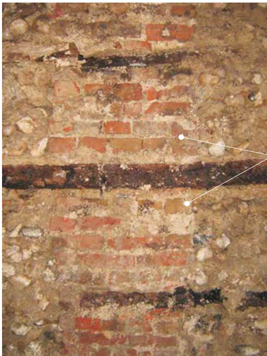
Plate 6 : The flush brick tie or stitching at the eastern end of the north elevation with timber plates
