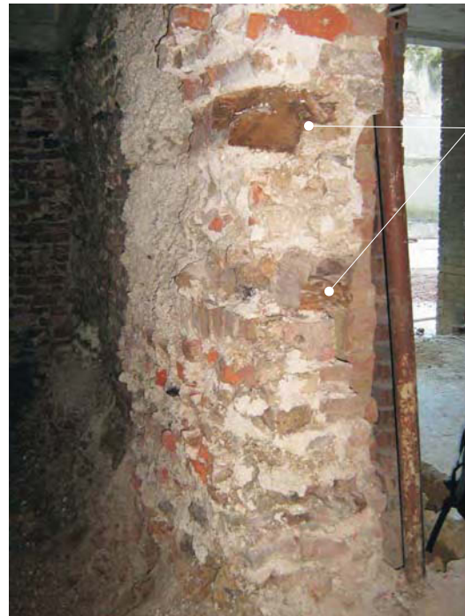
Plate 2: Section through the north wall created for modern access
