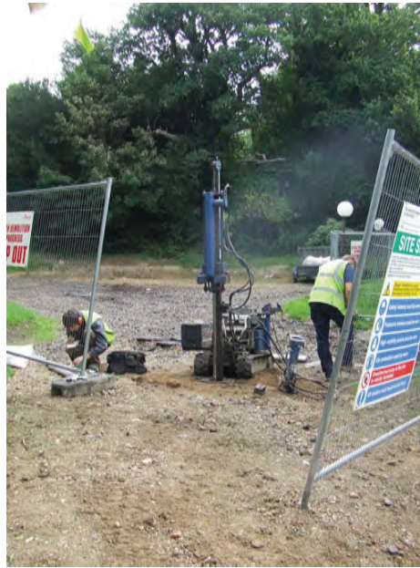
Fig. 4: Drilling the boreholes [1040]
