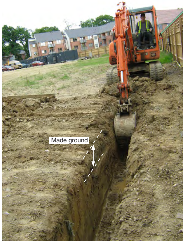
Fig. 3: Temporary Service Trench looking south-southeast
