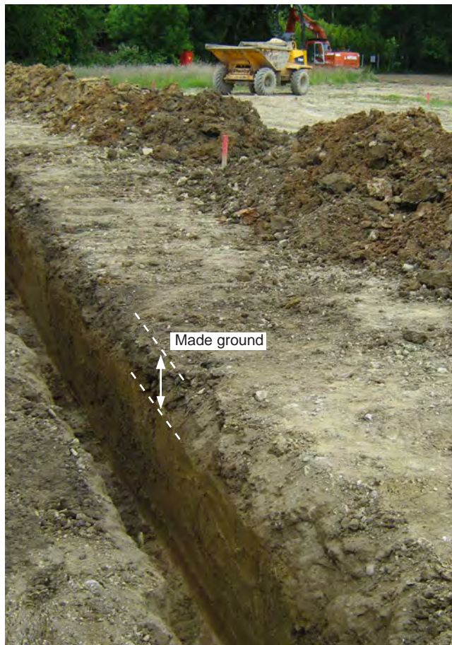
Fig. 4: Temporary Service Trench looking north-northeast
