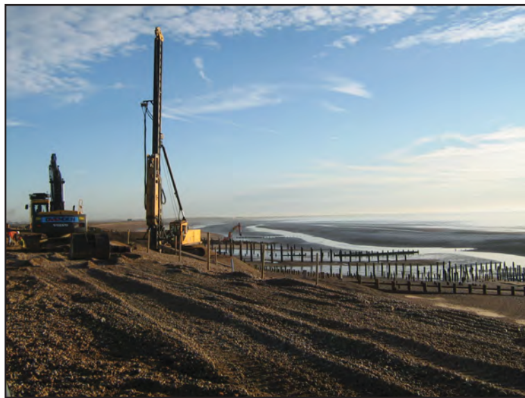
Figure 5: Start of piling on Groyne W6
