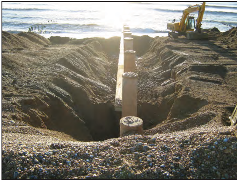
Figure 18: Excavations around Groyne W6
