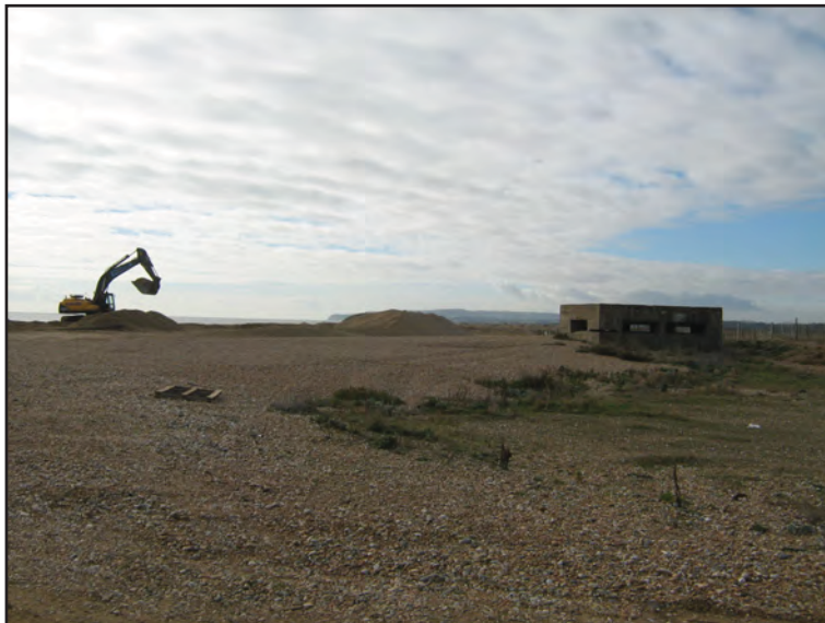
Figure 20: Shingle extraction works at The Nook, showing nearby pillbox
