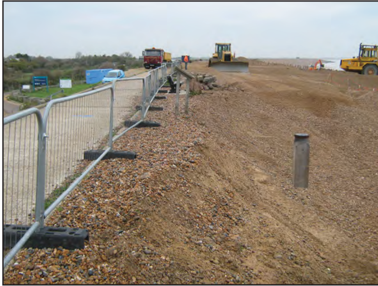
Figure 15: Work in progress along the sea wall north of Smeaton's Harbour
