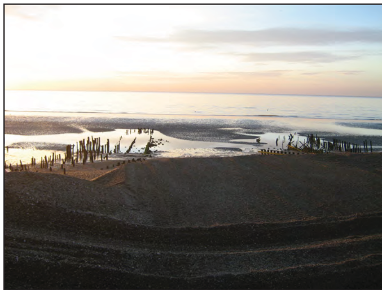
Figure 4: Smeaton's Harbour before piling commenced
