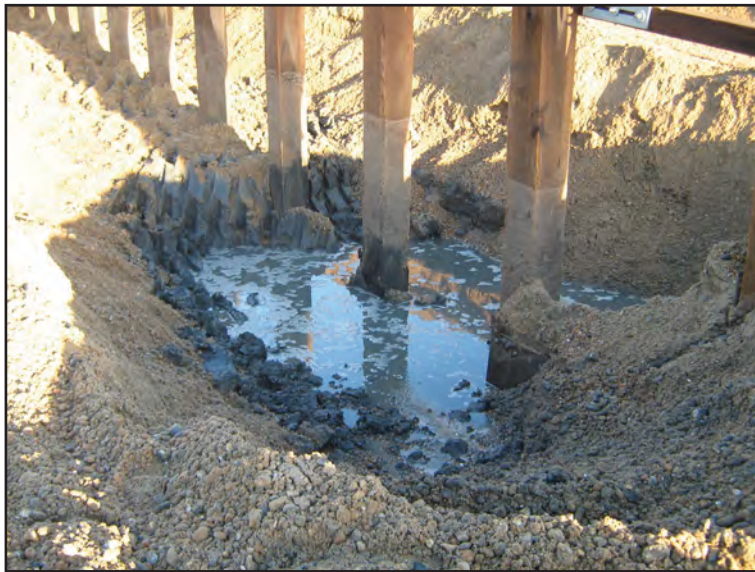
Figure 17: Excavations around Groyne W6
