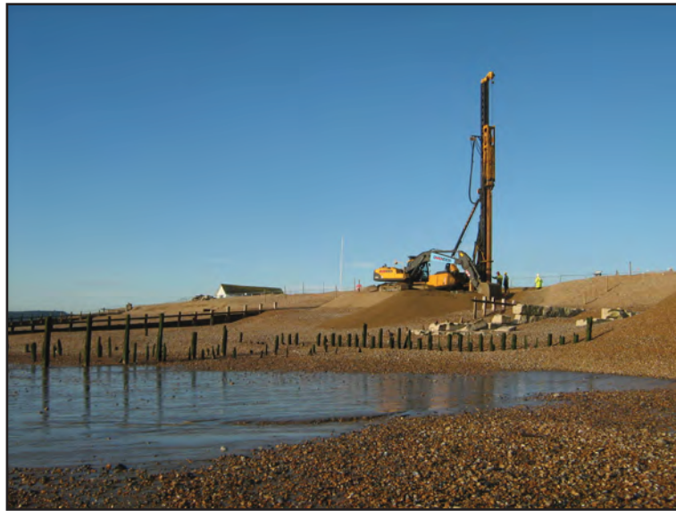
Figure 6: Piling on Groyne W6, showing East Pier of Smeaton's Harbour
