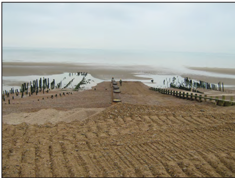
Figure 14: Groyne W6 between the two piers of Smeaton's Harbour
