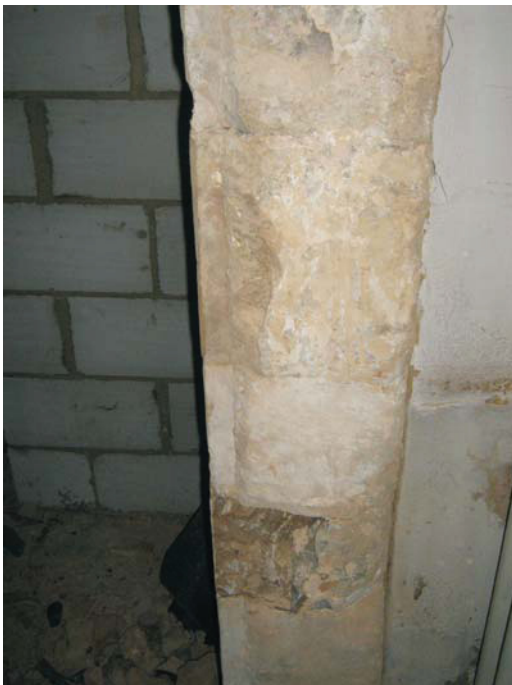
Figure 6: The rebated eastern edge of the doorway
