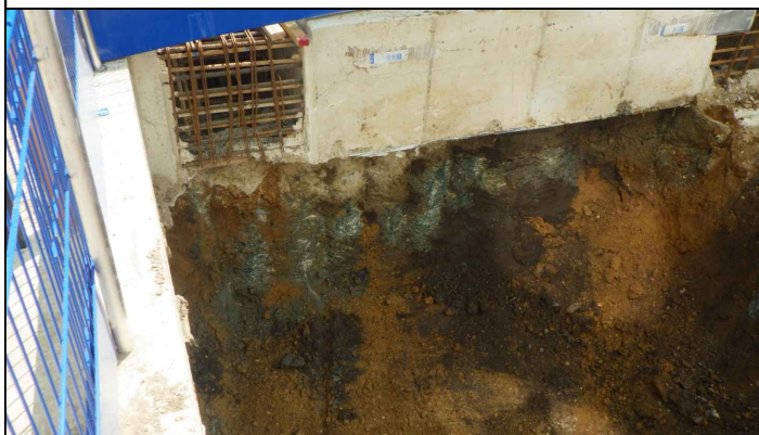
North-eastern corner of the site including drainage trench 104, looking south-east
