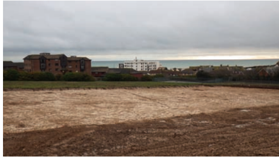
Photograph of the excavation area looking south west
