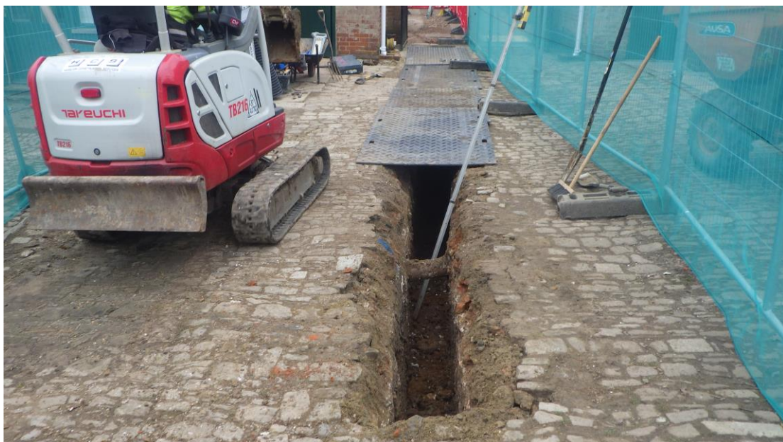
Courtyard excavations showing cobble surface [022]
