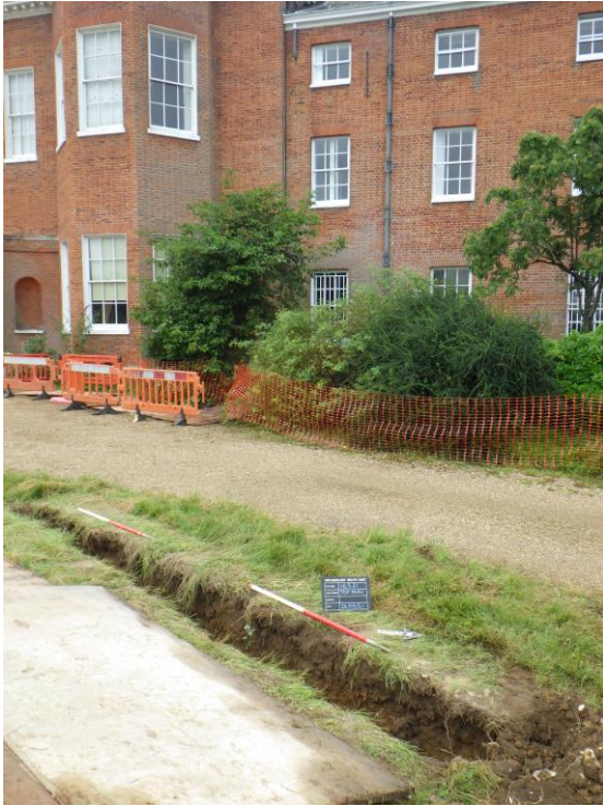
Service trench excavation adjacent to house
