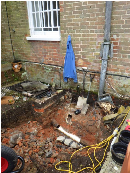
Service trench excavation next to house
