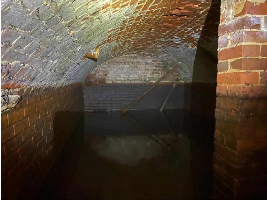
Brick vaulted chamber
