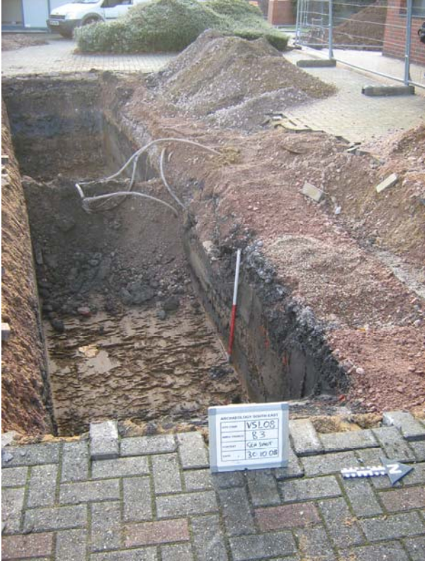
Fig 5: West facing shot of Trench B3
