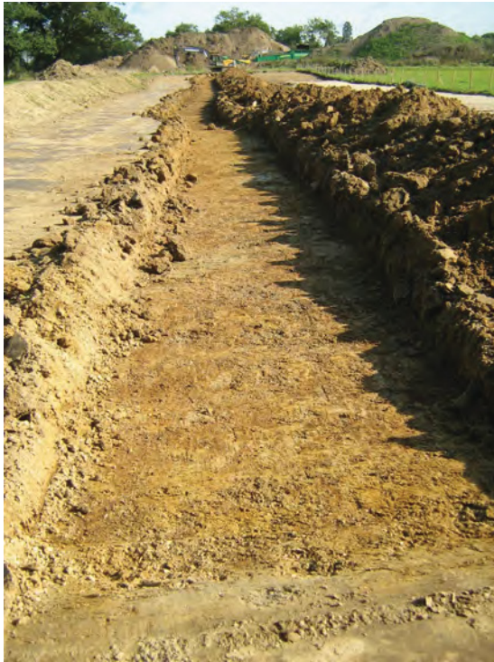
Fig. 3: East-facing shot of trench along route of pipe
