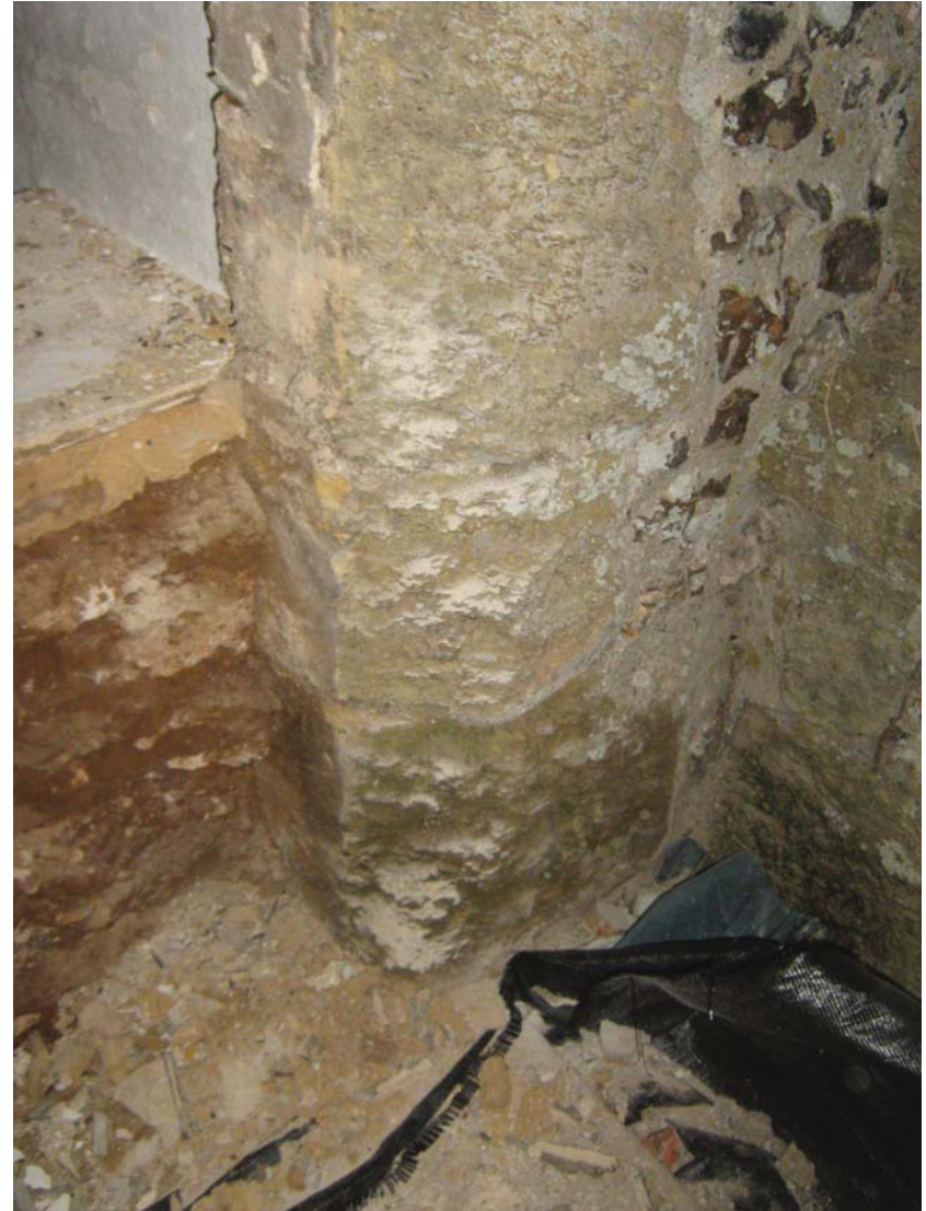
Fig. 8: The chamfer stop at the base of the eastern edge of the doorway
