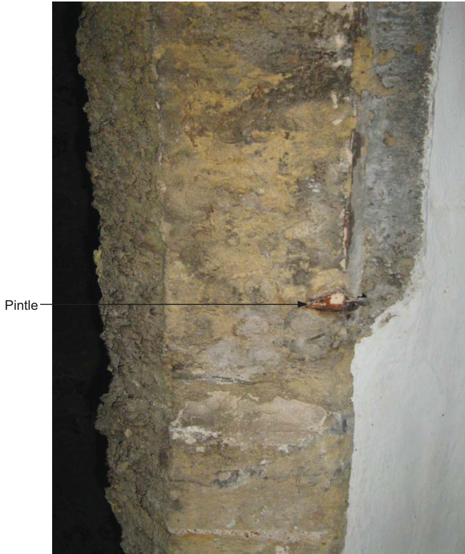
Fig. 9: The remains of the pintle on the west side of the doorway
