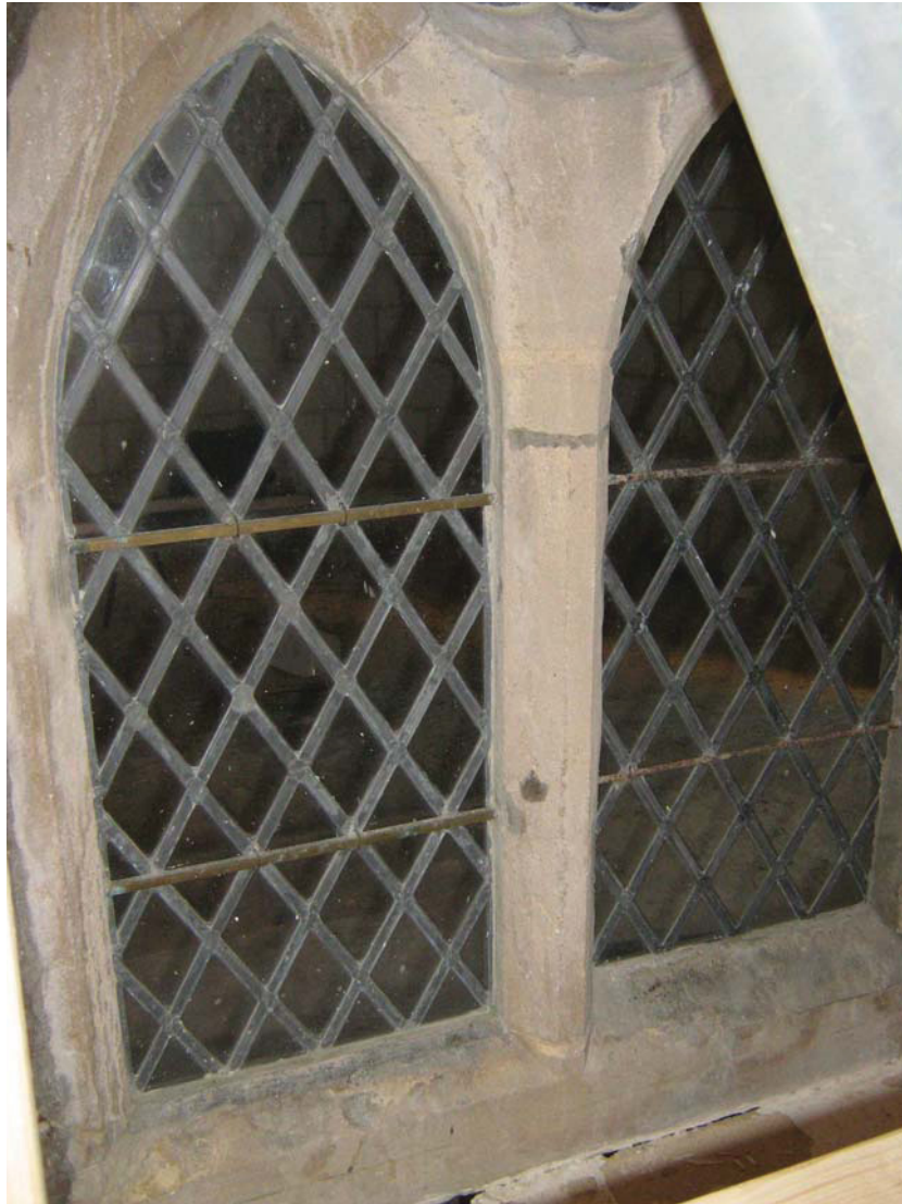
Fig. 11: Interior view of the inserted window still in situ
