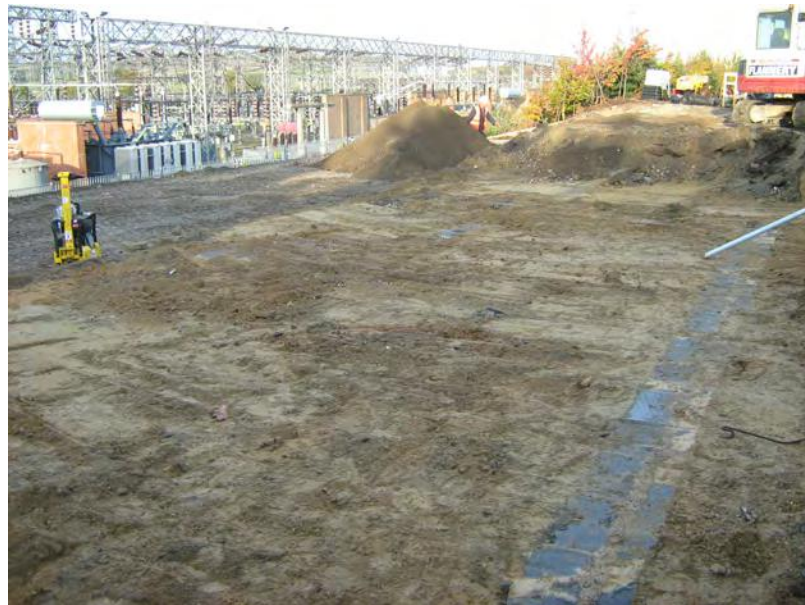
Fig. 5: Level strip before concrete laid for new offices and laboratory
