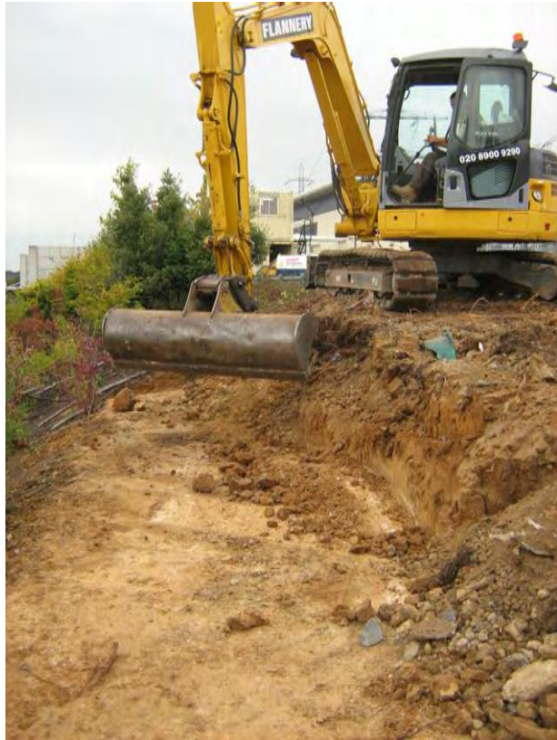
Fig. 4: Excavation in progress on the bank near the site entrance
