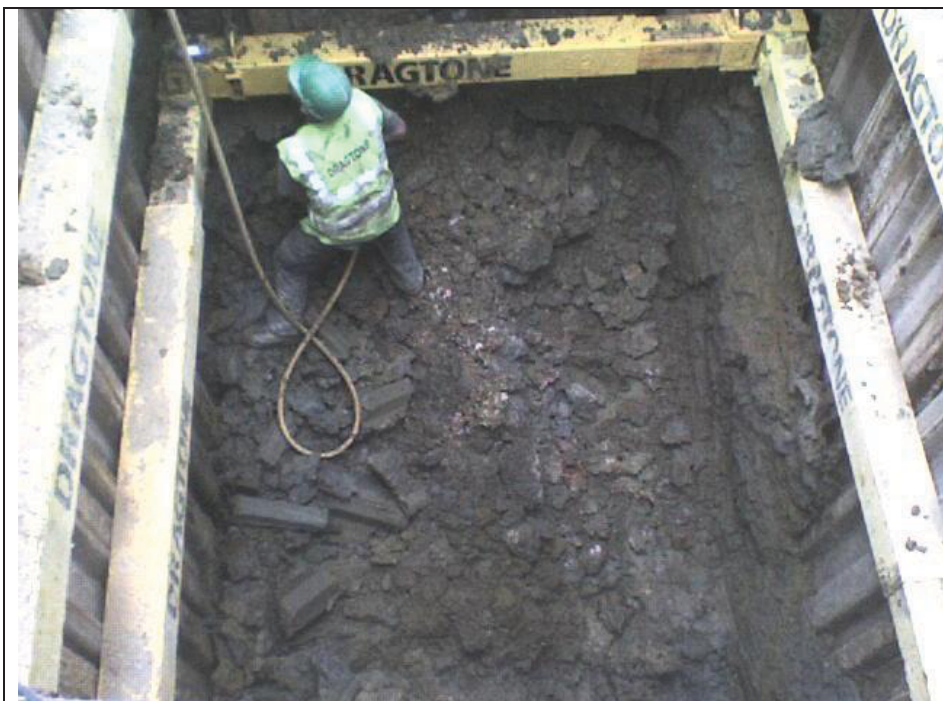
Figure 7: Exposure of Tertiary Beds underlying Head deposits in manhole 1, Lansdowne Road
