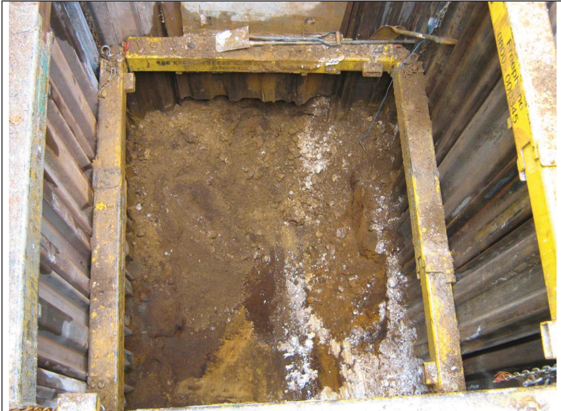
Figure 11: Exposure of Upper Chalk below Weathered Tertiary deposits at Wilbury Avenue, GTP3.
