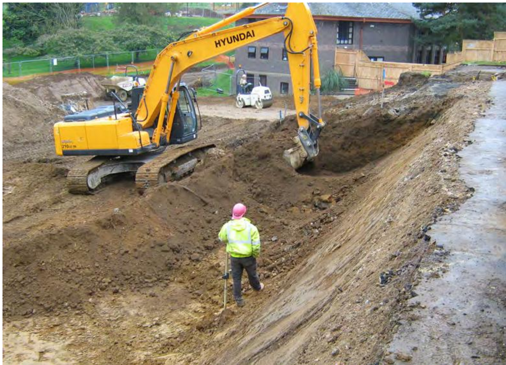
Fig. 4: Working shot of ground reduction, facing south-east
