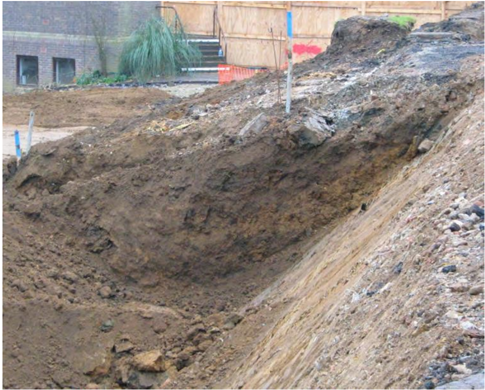
Fig. 5: North facing section of ground reduction
