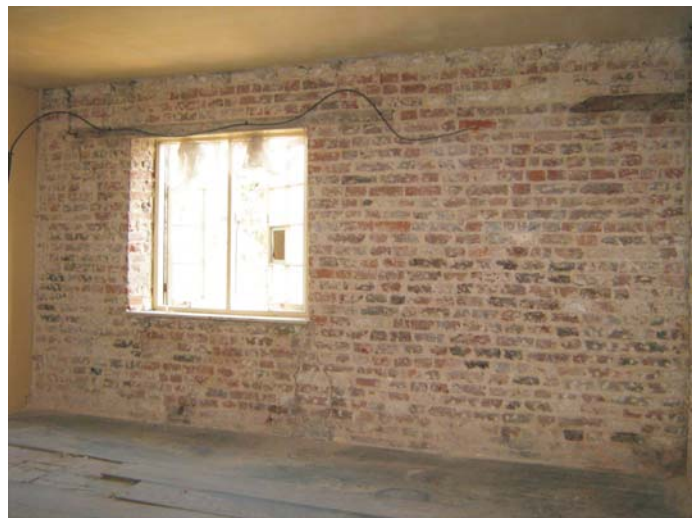
Plate 59: The north wall of bedroom 1
