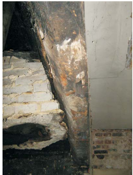
Plate 39: The bressumer over the fireplace in the living room with redundant mortises in the soffit
