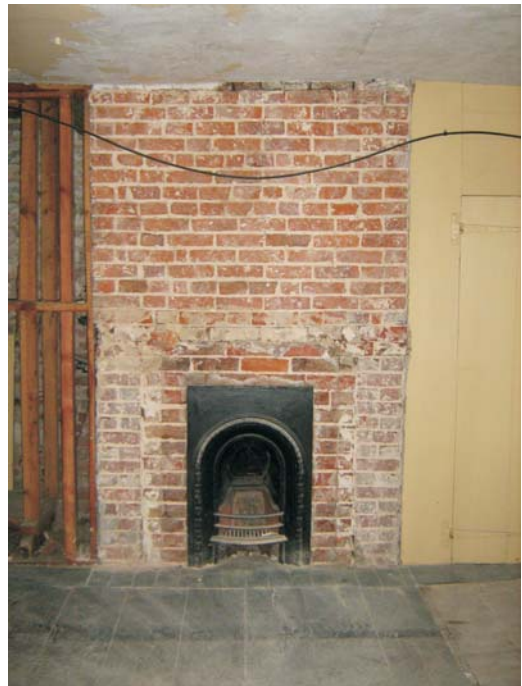
Plate 61: The west wall of bedroom 1 with in situ register grate
