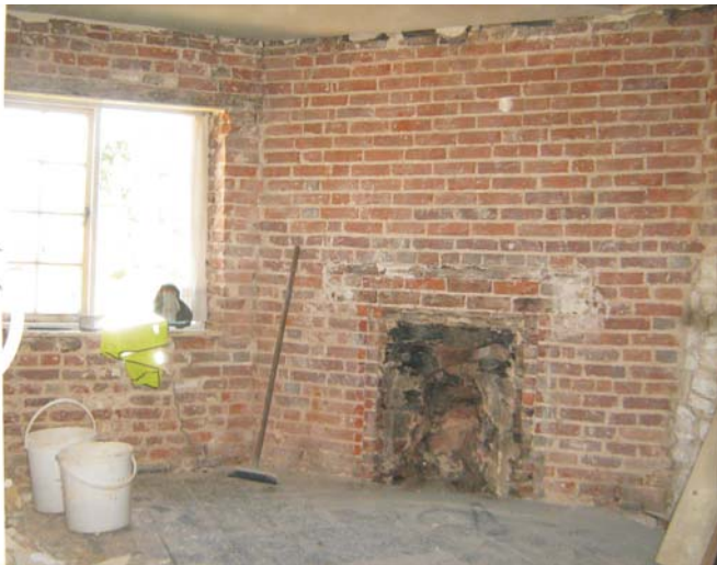
Plate 66: The north wall and the angle set fireplace in bedroom 2
