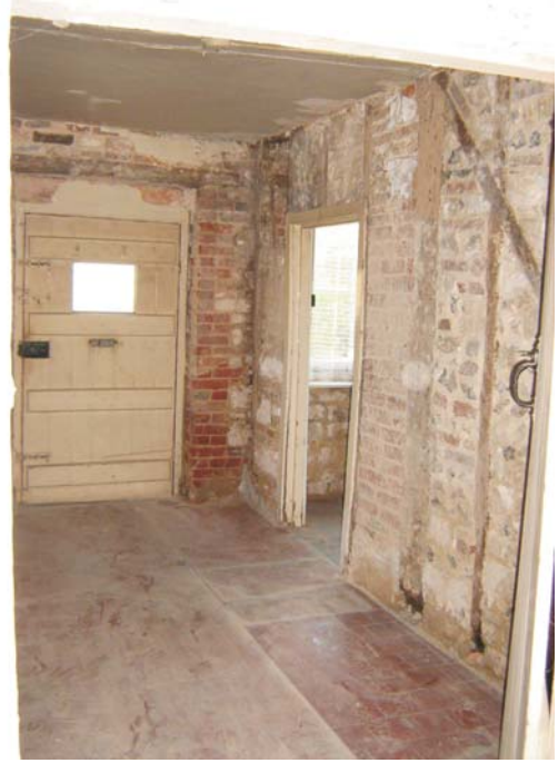
Plate 33: The timber frame partition wall between entrance hall and sitting room
