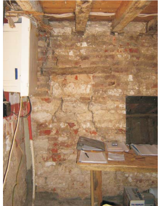
Plate 18: Detail of small blocked recess with timber lintel in the south wall of the kitchen. Also visible are the remains of the reed under-plaster ceiling above the junction box.
