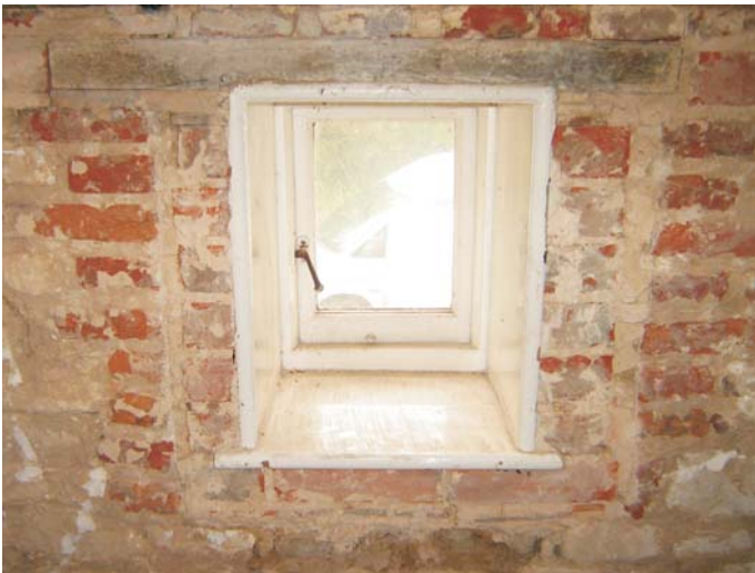
Plate 31: The reduced window opening within the bedroom 2 closet (store)
