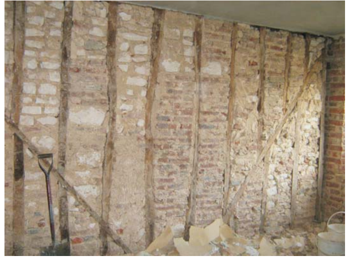
Plate 69: The west side of the timber framed partition between the bedrooms
