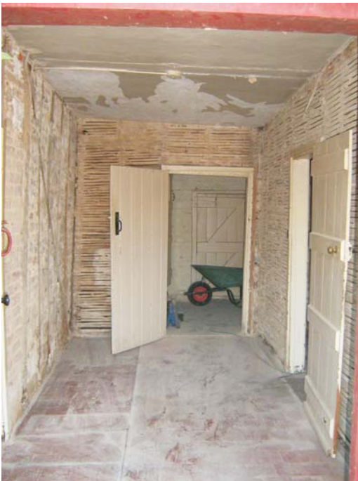
Plate 34: The south side of the entrance hall with quarry tile floor
