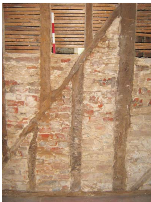
Plate 45: Detail of the timber framed south wall of the sitting room with in situ predominantly brick nogging to the lower part and the later laths visible on the bathroom side
