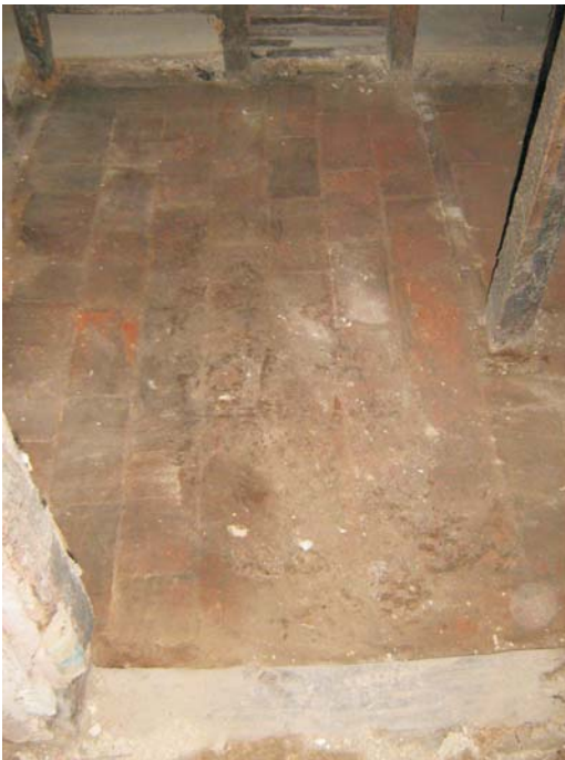
Plate 58: The brick floor of the under-stairs area
