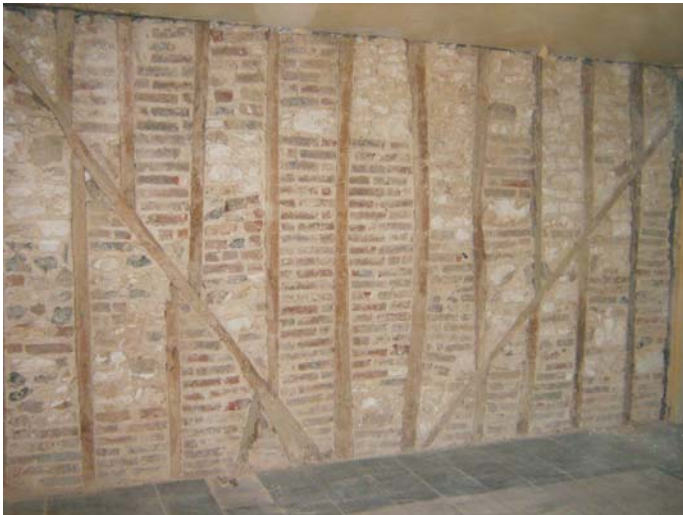
Plate 60: The east timber framed, brick and chalk in-filled partition wall between the bedrooms
