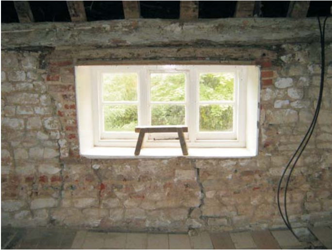
Plate 25: The west wall of bedroom 1 shows chalk block and brick construction
