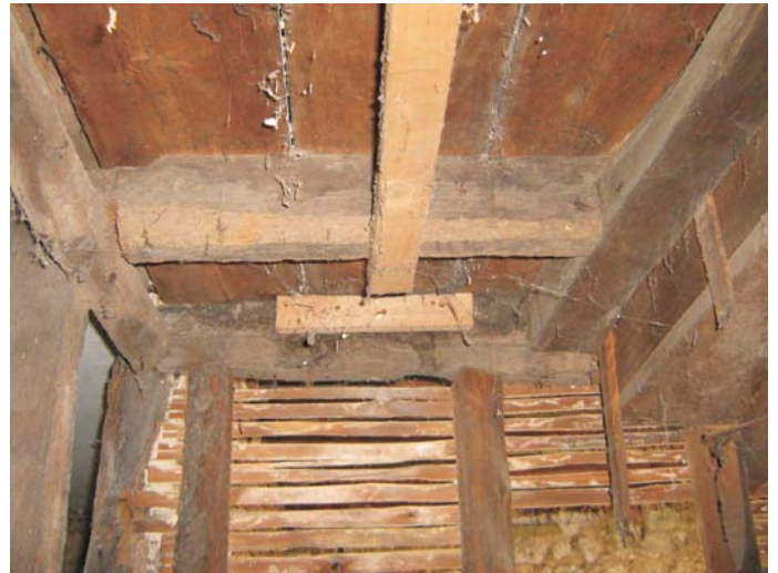
Plate 55: The underside of the staircase shows jointed joists to the south
