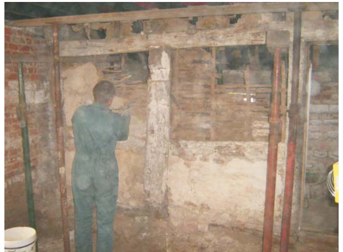
Plate 4: Stripping out of the south partition wall in progress - October 2008
