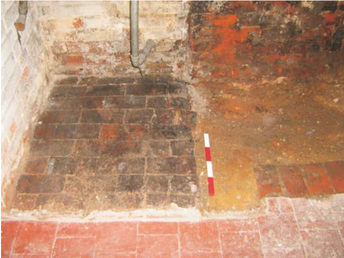
Plate 40: The hearth of the fireplace still in situ where the south cupboard had been added
