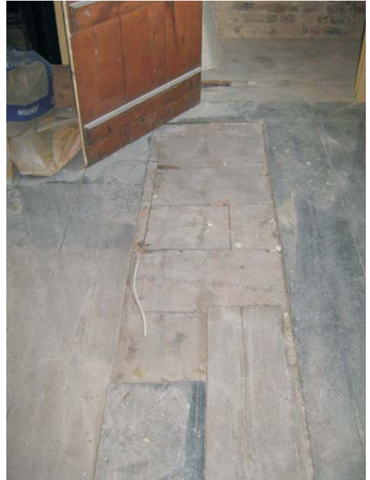
Plate 65: Detail of the two layers of floorboards in bedroom 1
