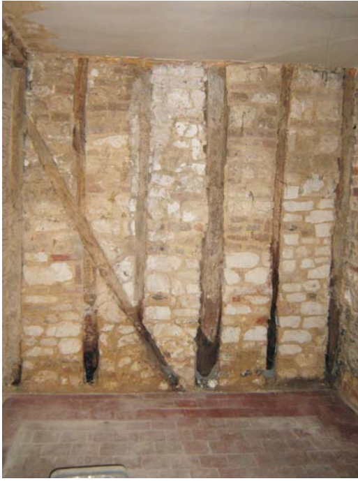
Plate 36: The timber frame south wall of the living room
