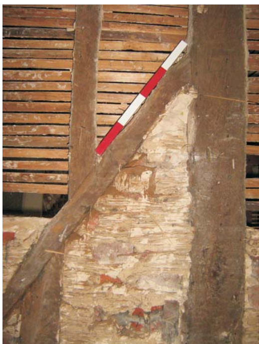
Plate 46: The south wall of the sitting room detail of the plaster in a reed matrix overlying the brick nogging
