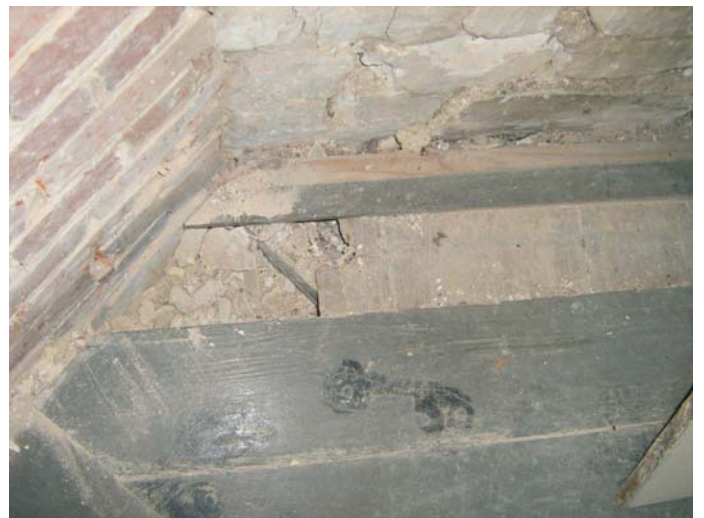
Plate 71: Detail of the two layers of floorboards in bedroom 2
