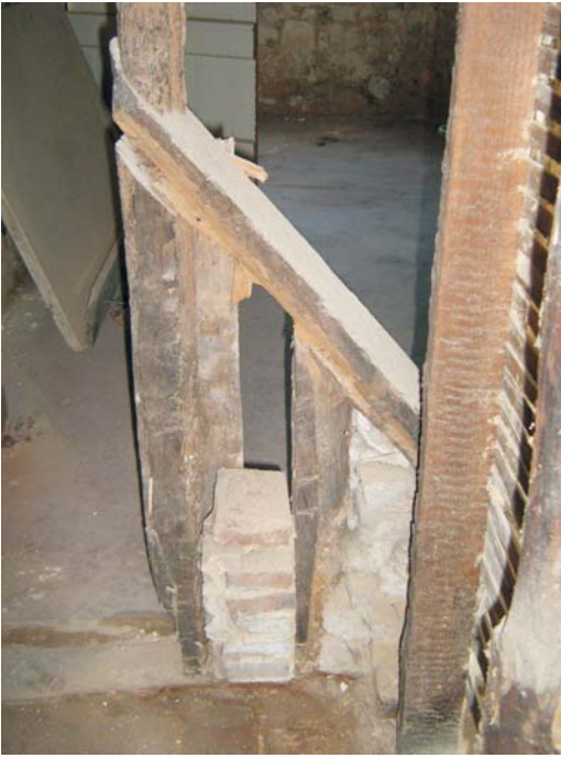
Plate 56: Truncated strut at the base of the doorway in the south partition wall of the sitting room
