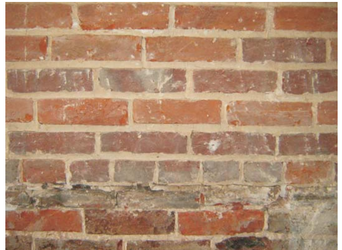
Plate 67: Detail of the brickwork of the chimney breast
