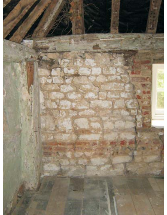
Plate 26: Detail of the south side of the window in the west wall of bedroom 1 - insertion rather than reduction of original opening as shown by the brickwork
