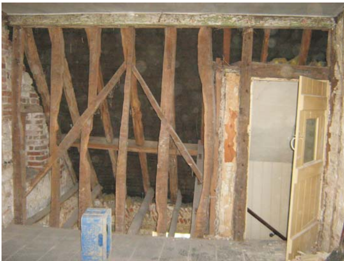
Plate 70: The timber framed south wall of bedroom 2
