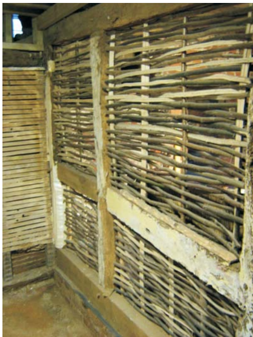
Plate 7: The south wall with replacement in-fill in situ - January 2009
