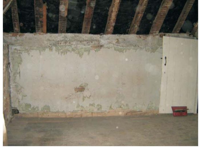
Plate 30: The timber framed south wall of bedroom 2 with the plaster in situ
