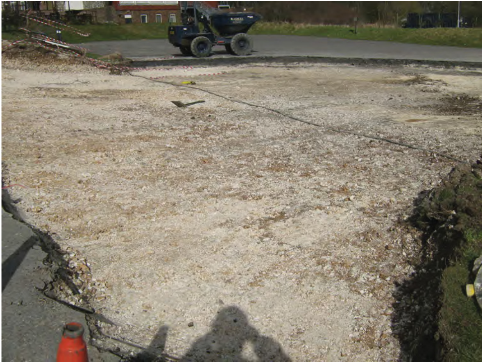
Fig. 3: Area 1.1 under excavation, looking north-east
