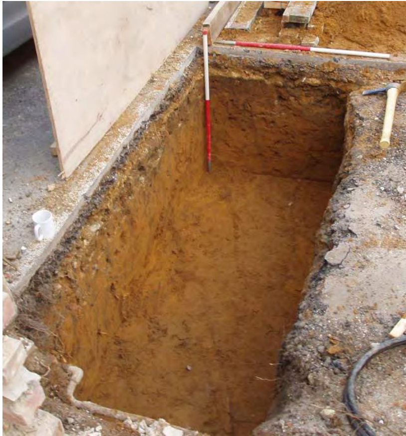
Plate 1: Photograph showing the western footing trench, looking north
