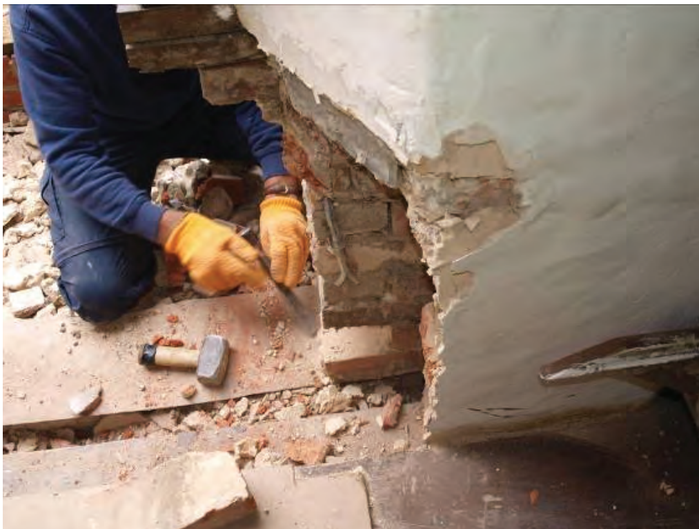
Figure 6: The lead lining to the foundation of the wall exposed after demolition
