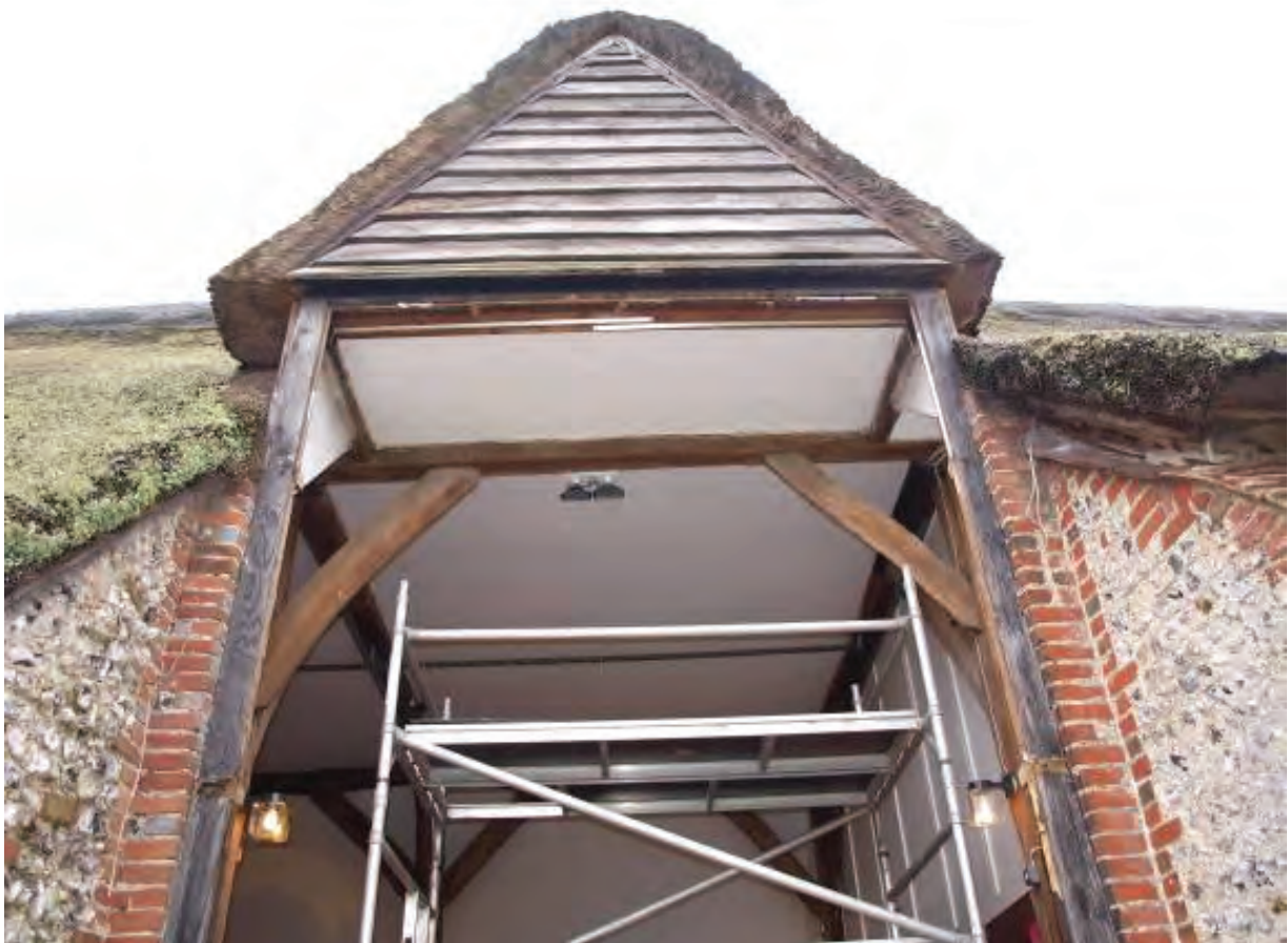
Figure 3: Detail of the top of the opening after the removal of the window.
