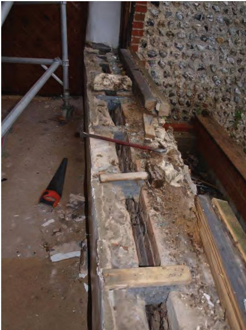
Figure 5: Detail of the wall construction from the top, just prior to demolition. View shows the two skins and the breeze block bridges.
