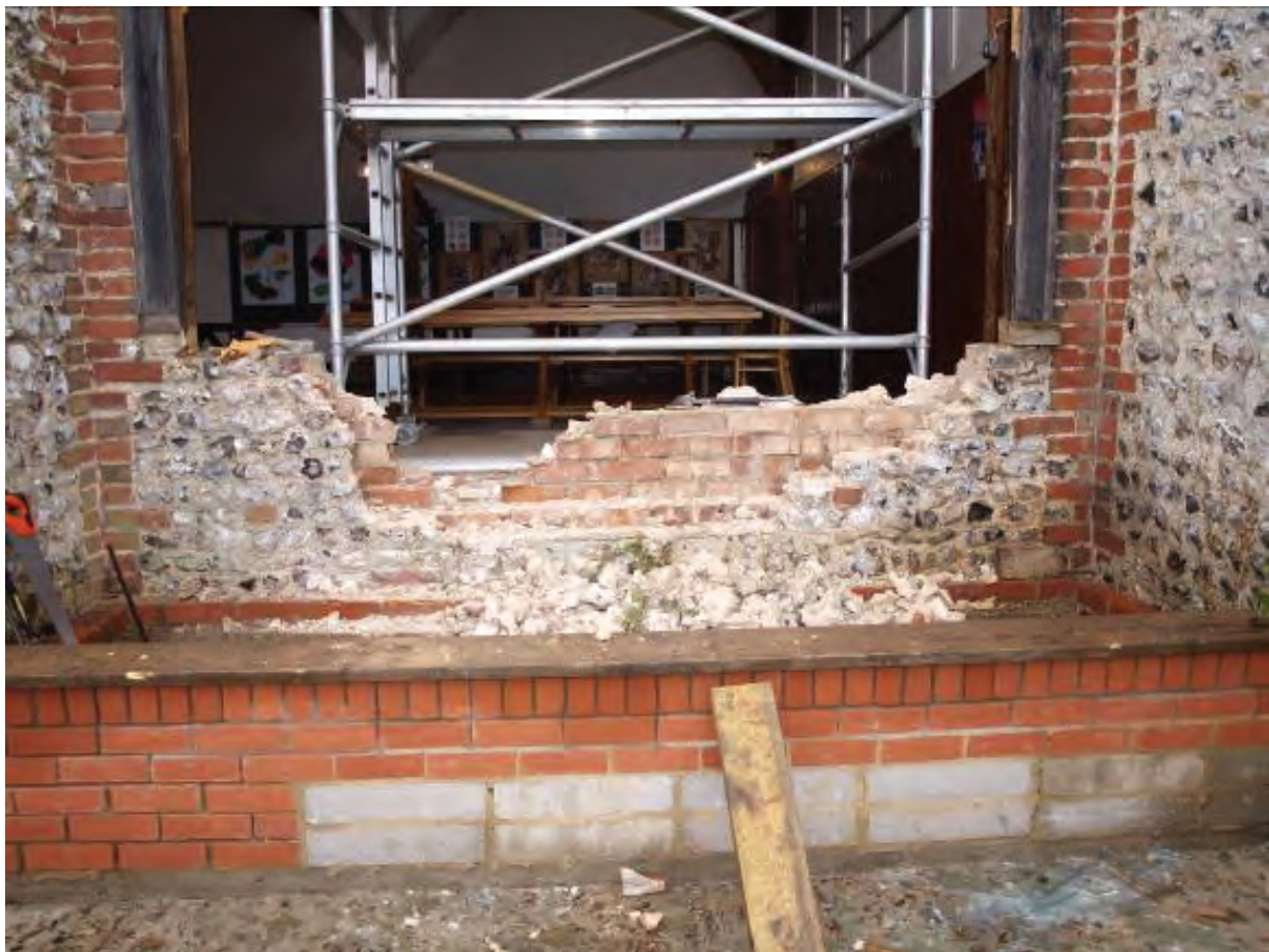
Figure 4: view of the wall during demolition showing the flint facing of the outer (northeastern) skin and exposing the brickwork of the inner (southwestern) skin.
