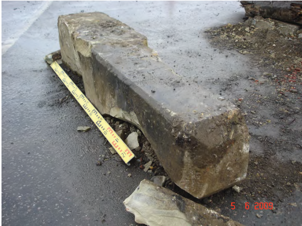
Fig. 7: The milestone showing chamfered corners and top
