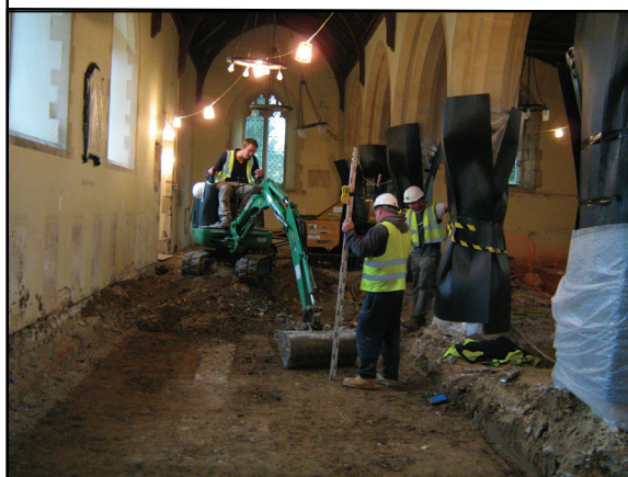
Fig. 3.2: Ground reduction (south aisle)
