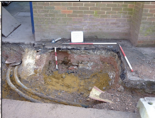
Fig. 4.4: Test pit 4, facing south
