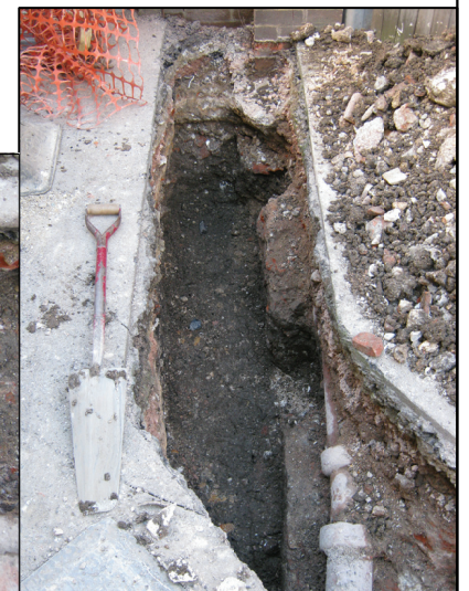
Fig. 7.2: Wall foundations 5/013 and 5/014
