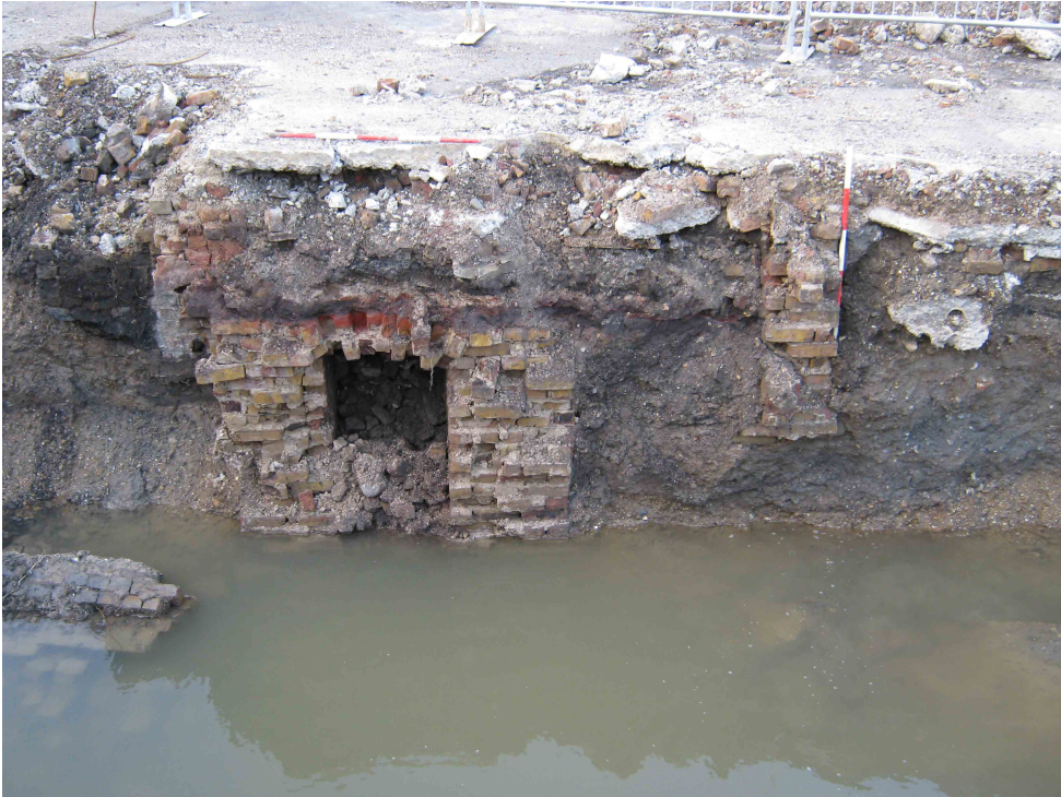
Fig. 9 South Section showing culvert 009 and other masonry features
