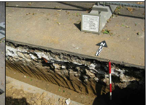
Fig. 3.2: Wall footing 008, looking north
