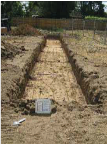
Fig. 6.1: Trench 1 looking south-east
