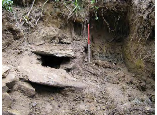
East side of culvert, looking west
