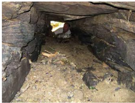
Culvert internal facing west
