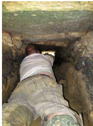
The joys of culvert clearance
