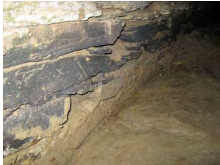
Culvert south wall
