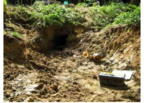
Culvert east end facing west
