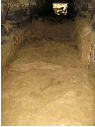
Culvert base facing west
