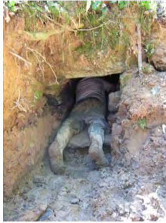
Culvert clearance underway
