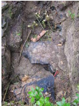
East end of culvert
