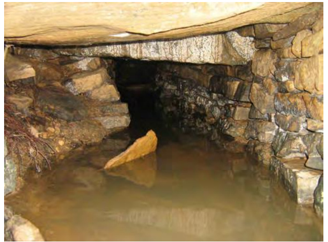
Interior of Strawberry Wood culvert
