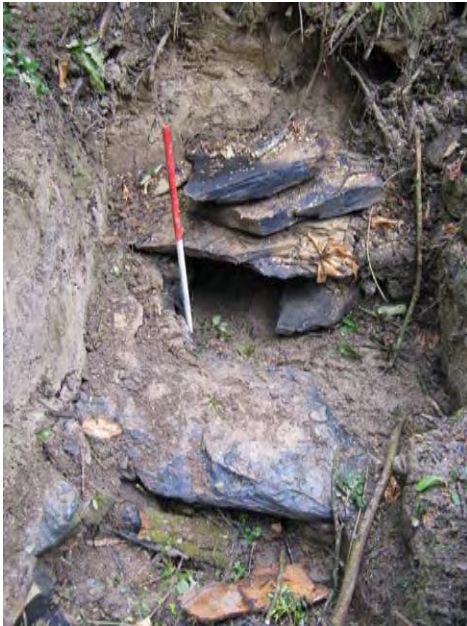
West side of culvert, looking east
