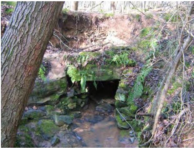
Strawberry Wood culvert before restoration
