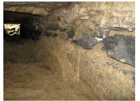
Culvert north wall
