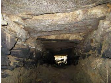
Culvert roof facing west
