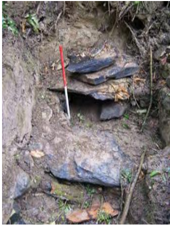
Culvert facing east
