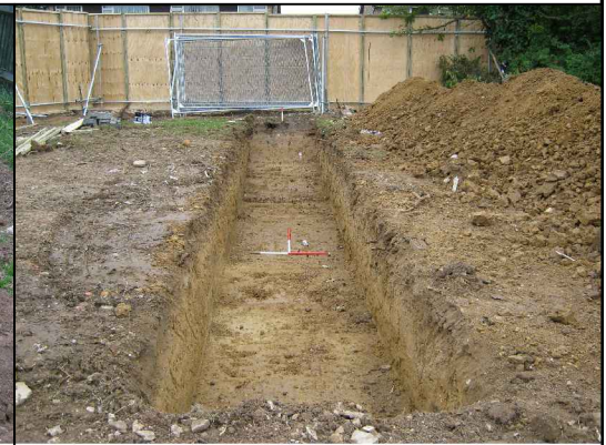
Trench 4 facing south
